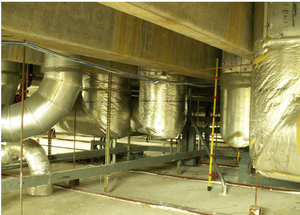
Photo B-6 Interior Service Module Showing ducts to interstitial service zone from penthouse
