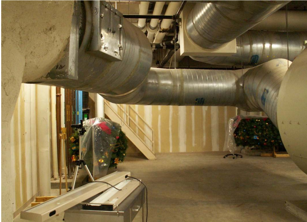
Photo B-5 Service Bay Showing crossovers of ducts and piping
