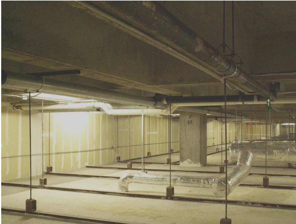
Photo B-1 Interstitial Service Zone Near end of main runs
