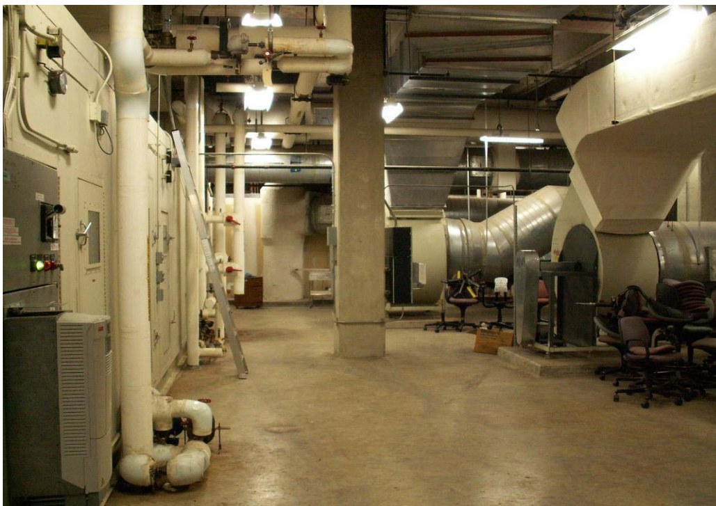
Photo B-4 Typical Service Bay
