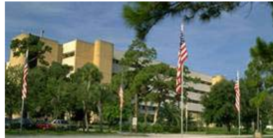
VA Medical Center Bay Pines, FL, 1983
