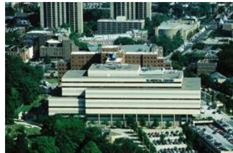
VA Medical Center Philadelphia, PA, 1994 (not VAHBS, used interstitial space)
