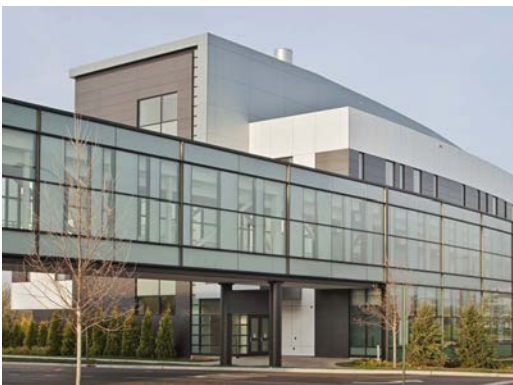
Figure 4.4.3: An enclosed skyway connects two buildings, allowing views of the exterior during passage. Health and Science Center, College of DuPage. Glen Ellyn, Illinois.
