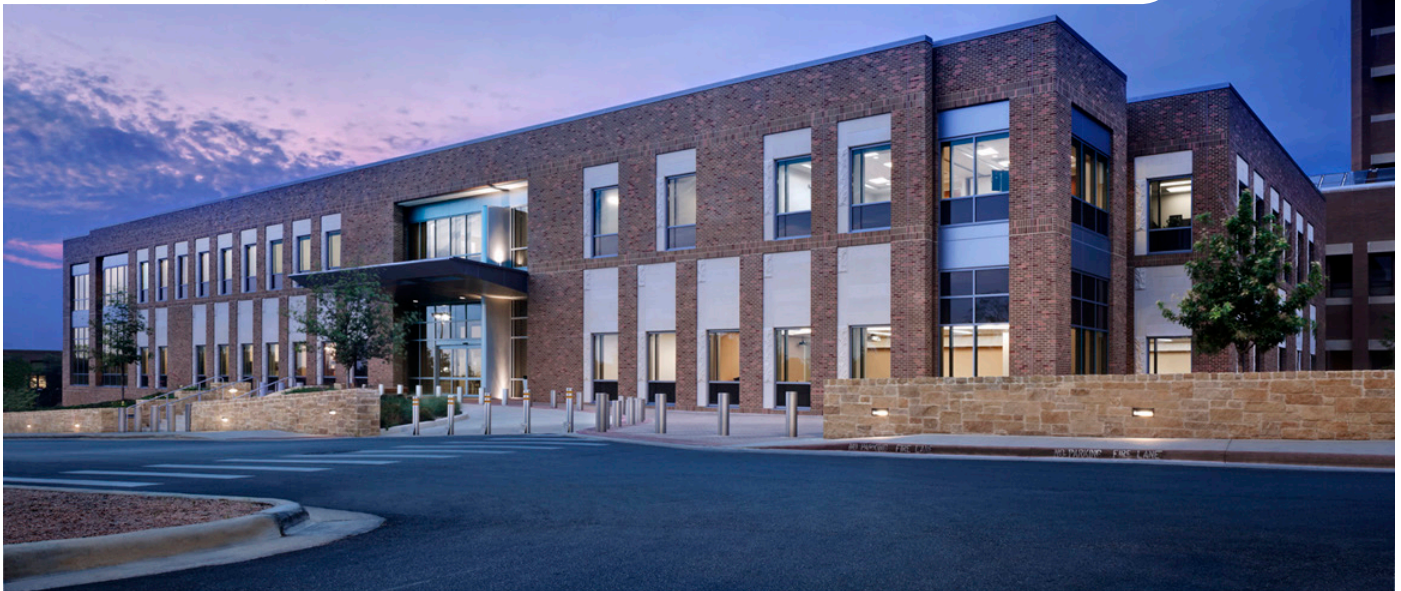
Figure 3.4.1: Regional building materials such as brick, plaster, and fieldstone are applied to the building and boundary fence. Polytrauma Rehabilitation Center, Audie L. Murphy Memorial VA. San Antonio, Texas.
