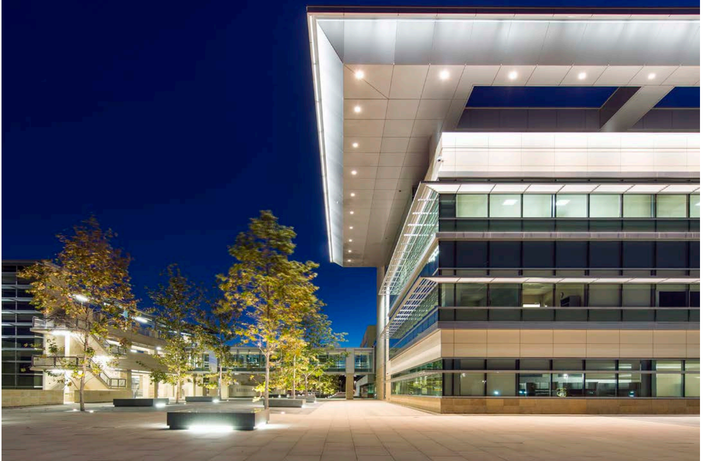
Figure 5.1: Naval Hospital at Camp Pendleton. Camp Pendleton, California.
