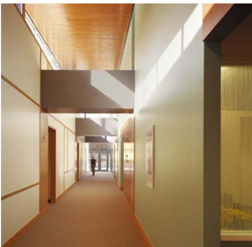
Figure 4.4.4: This one-story building element with clerestory allows natural light to penetrate a double-loaded corridor. UW Cancer Center Johnson Creek. Madison, Wisconsin.
