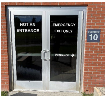
Figure 1-2 (Above) Inconsistent and conflicting information negatively impacts wayfinding and confuses visitors. Seen here: "Not an Entrance" on the door and "Entrance 10" on the sign next to the door."
