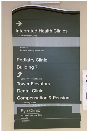
Figure 1-5 (Above) This directional sign has multiple issues. Message panels are missing or broken, some text is too small, and arrow placement is confusing.
