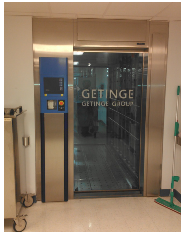
Figure 6: Automated Cart Washer (SPS)
