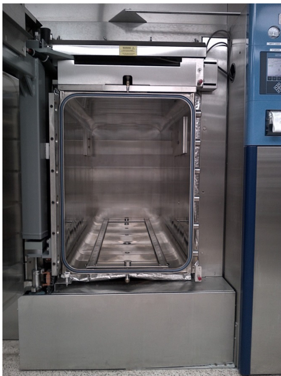
Figure 13: Front Loading Steam Sterilizer (SPS)
