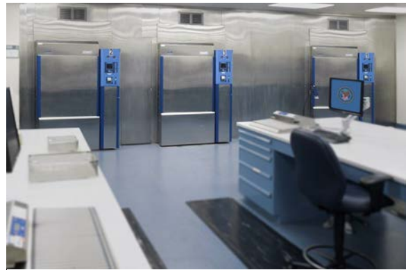
Figure 11: Steam Sterilization Room (SPS)
