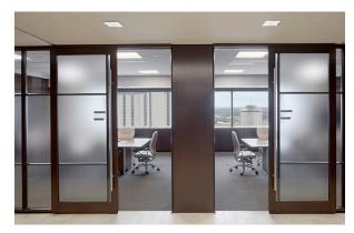
Figure 5.1-8 Example of Modular Wall System
