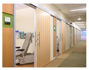
Figure 5.1-11 Sound-Proofed Wall and Door System \*Courtesy of CollinsWoerman Architects
