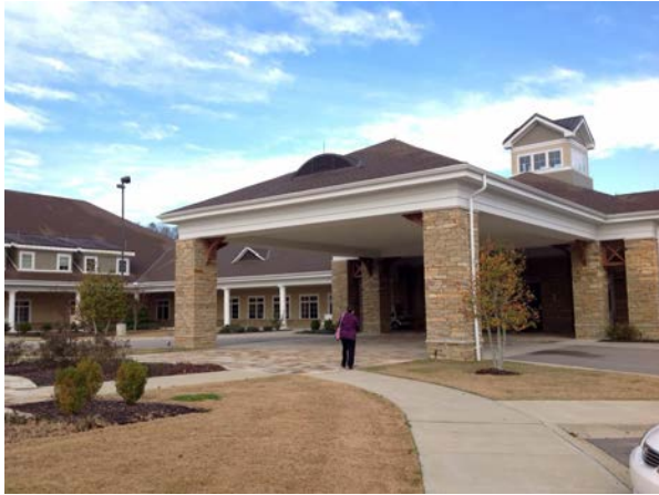
Figure 5.60 Photo Position A
