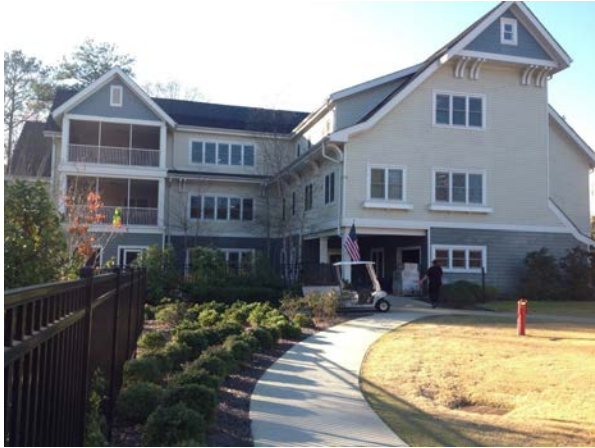
Figure 5.65 Photo Position A
