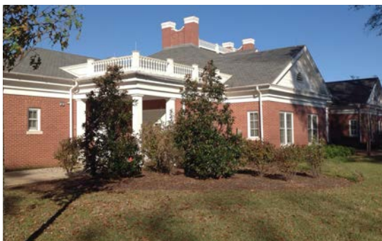
Figure 2.14 Landscape buffer at the Tuscaloosa, AL CLC.
