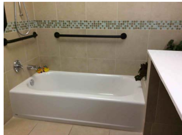
Figure 5.104 Photo Position E
