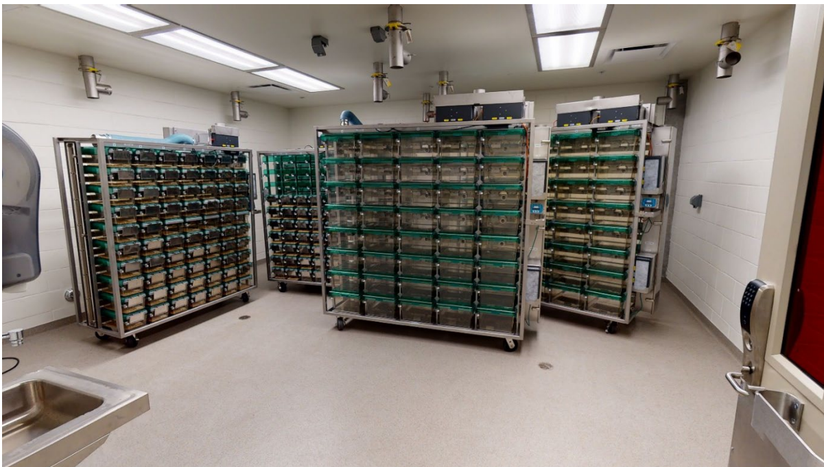
Image A.19 A Small Animal Holding Room at the New Orleans VAMC R&D Facility contains height adjustable ventilated cage racks, both single-sided and double-sided, which can be placed against a wall or freestanding in the middle of the room, respectively. The room also has exhaust vent pipes to evacuate dander and other particles.
