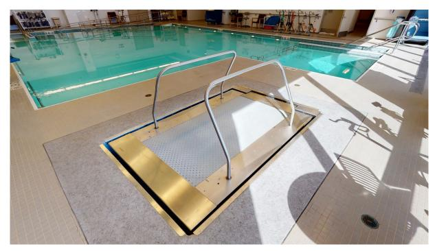
Figure 32 The AT Treadmill Pool at the New Orleans VAMC includes jets for resistance and cameras to observe underwater motion.
