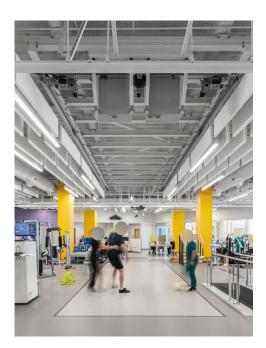
Figure 1 A two-rail, four-cable patient lift system is demonstrated at the Sheltering Arms Institute in Richmond, VA. (Photo courtesy of HDR © 2021 Quentin Penn-Hollar)
