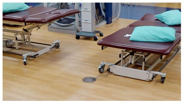
Figure 2 The Open Treatment Area at the Orlando VAMC PMR Svc, which is shared by PT and OT, incorporates outlets throughout the floor to power exercise and therapy equipment.
