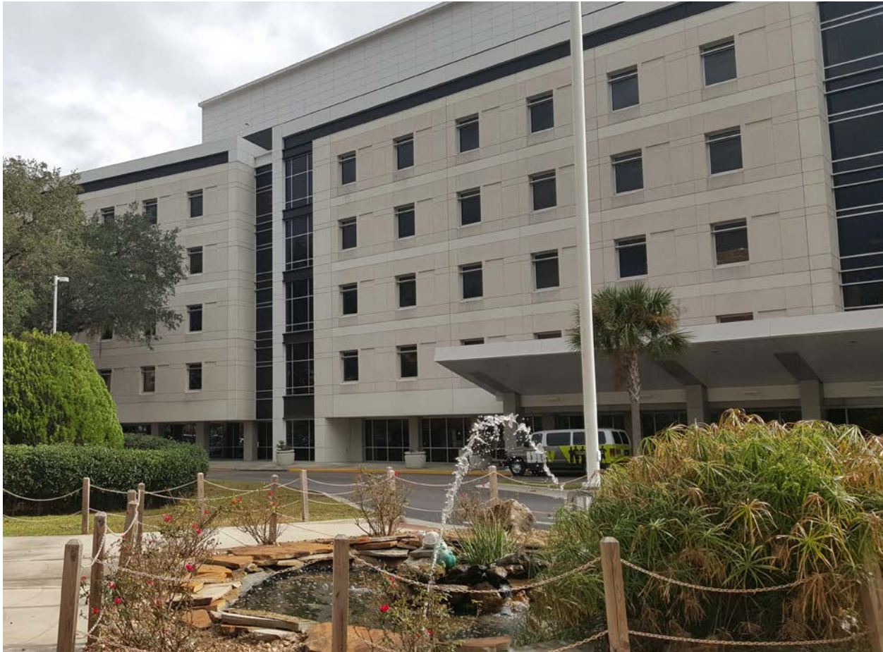
Figure 5.72 Main Entry of Malcom Randall VAMC
