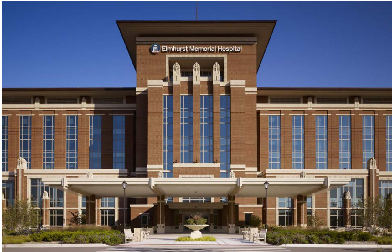
Figure 5.30 Main Entry of Elmhurst Memorial Hospital
