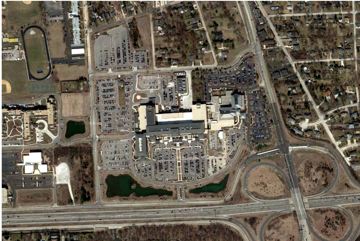
Figure 5.29 Aerial of Elmhurst Memorial Hospital
