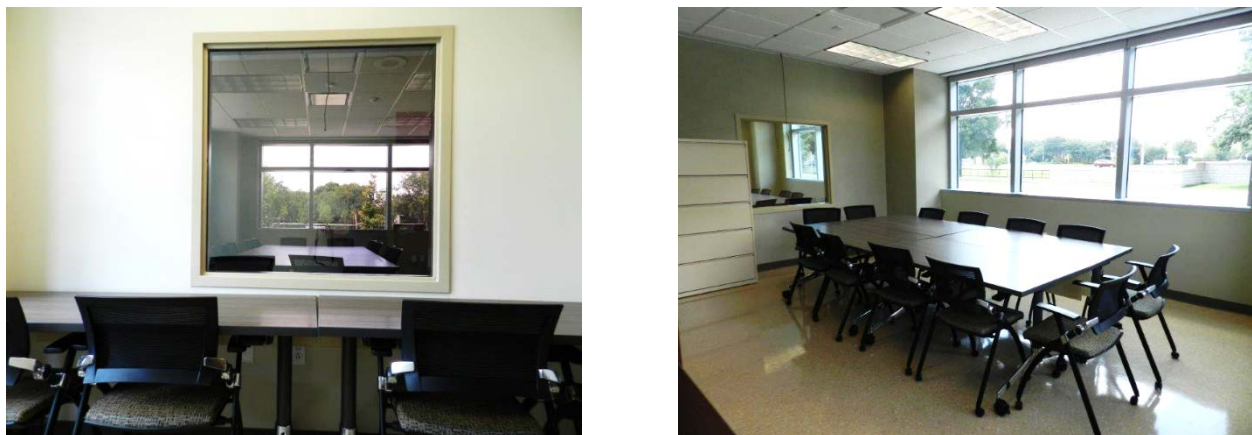
Figure 2.2.3.6.a: One-way mirrored window from viewing room to group therapy room, VA Tampa Primary Care Annex
