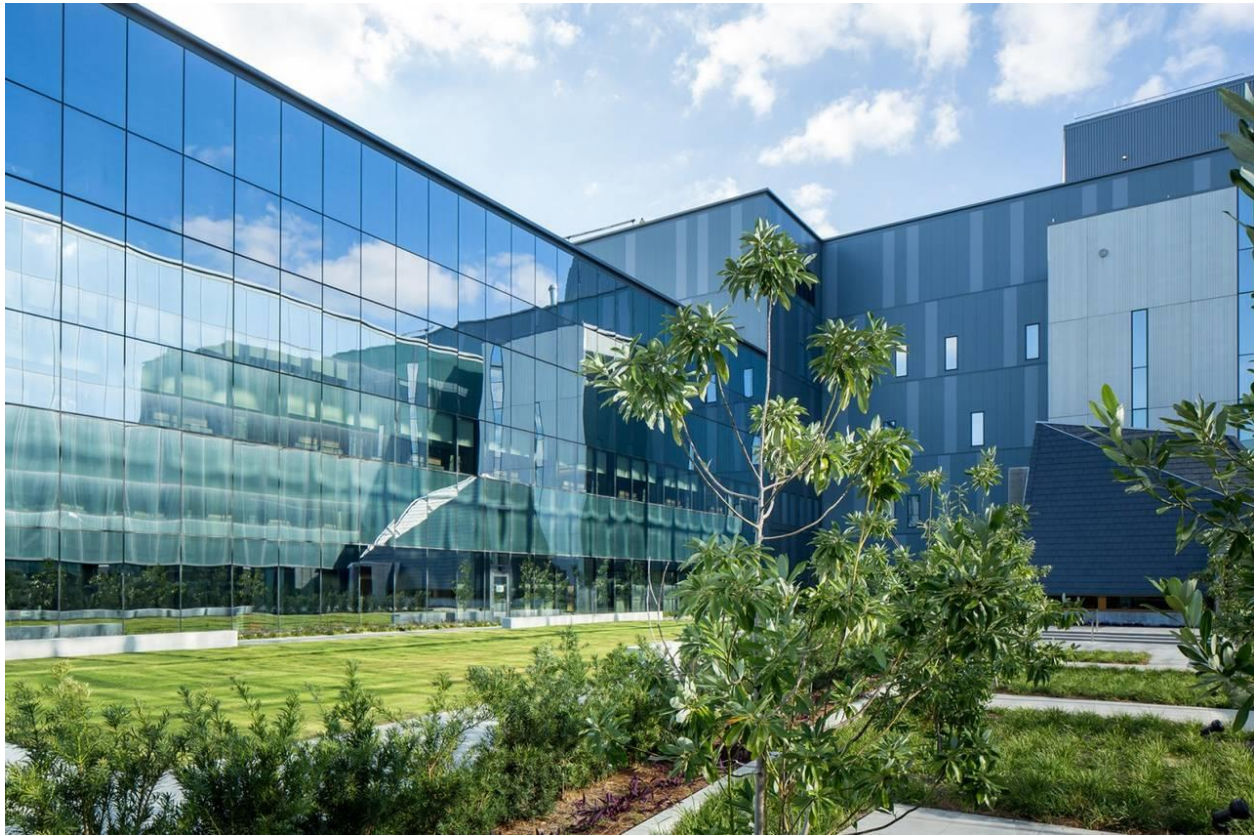
3.1 New Orleans VA Medical Center Exterior
