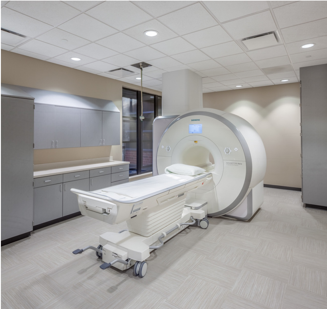
Figure 2.7.3.9: Example of an MRI Scanner Room (Image used with permission from RAD-Planning)
