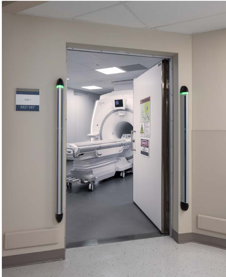
Figure 2.7.3.8-2: Example of door to MRI Scanning Room with ferromagnetic detection system flanking the doorway to Zone 4. (Image used with permission from RAD-Planning)
