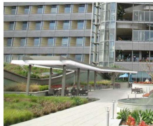
Figure 4.6.4: Covered rooftop garden area with multiple seating options, including tables for eating. Palomar Medical Center. Escondido, California.
