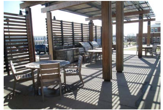
Figure 3.6.2: Outdoor barbecue and seating area. USO Warrior and Family Center. Ft. Belvoir, Virginia.
