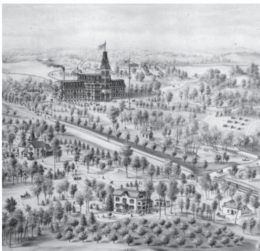
Figure D.14: Aerial rendering of Milwaukee Soldiers Home campus including therapeutic gardens, gazebos, and ponds. Milwaukee, Wisconsin.
