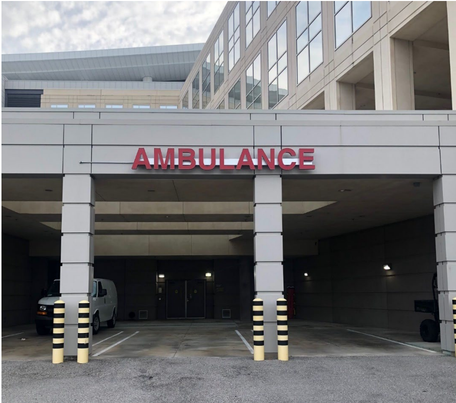
EMS / Ambulance covered entry point.
