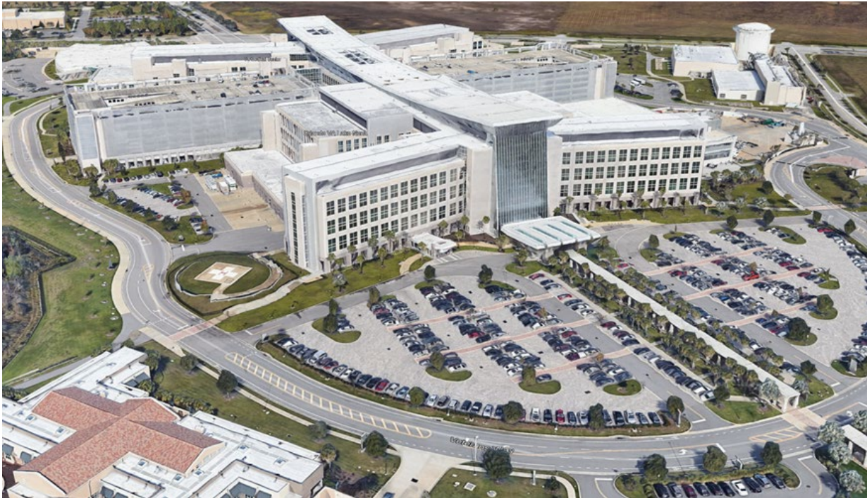
Orlando VAMC - Aerial View looking to the North at Walk-in Entrance.
