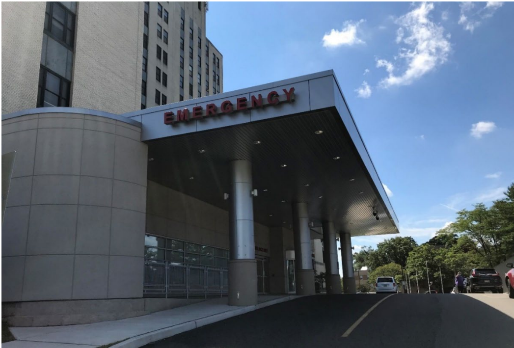
Drive through entry canopy for both EMS / Ambulances and Walk-in patient drop offs.
