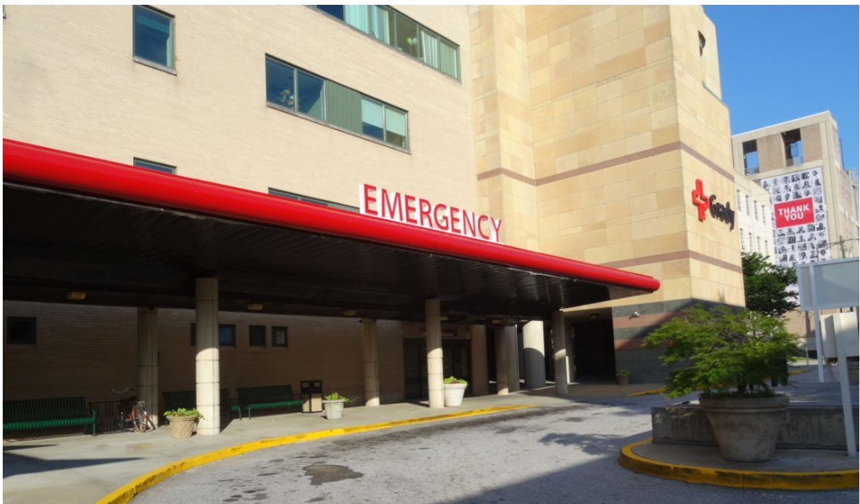
Photo of covered EMS / Ambulance drop off area above.
