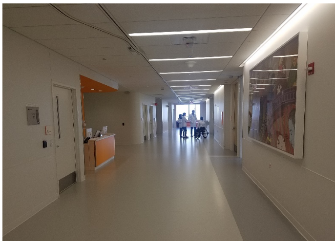
Extra wide patient corridors to accommodate wheelchairs and lifts
