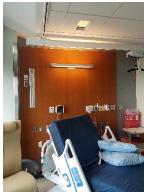
Patient bed with lift track and headwall.
