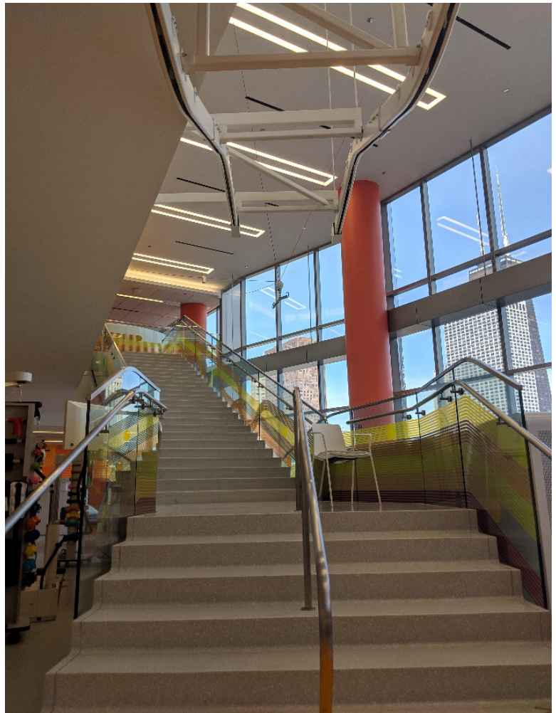
Exercise stairs are provided as a monumental stair, with daylight, views, and multiple overhead lift/support systems.
