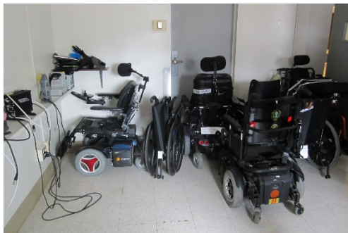
Space and circuits for charging powered wheelchairs are provided in storage room with supplementary ventilation.
