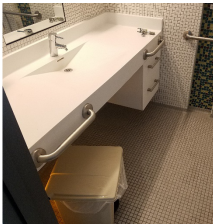
Customized integral sink is intended for ease of use and cleaning.
