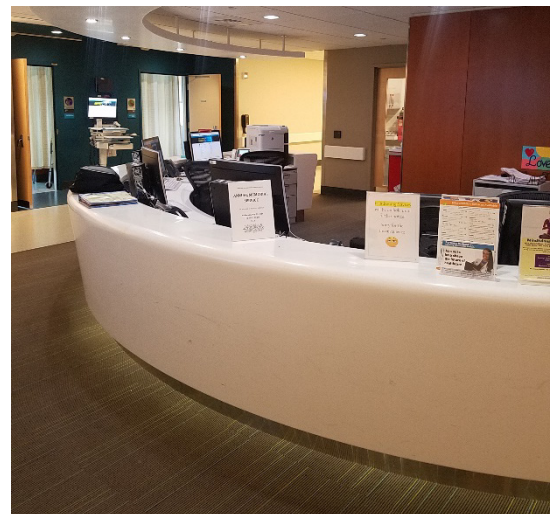
Central nurse station for visual control and greeting. Counter height shown may not be ADA Compliant.
