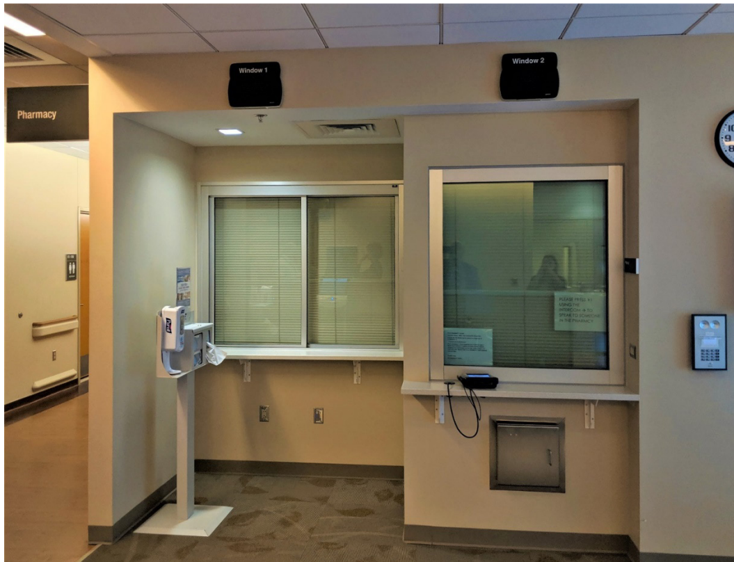
Figure 2.10 Rocky Mountain Regional VAMC SCI/D Pharmacy, with ABA pass through
