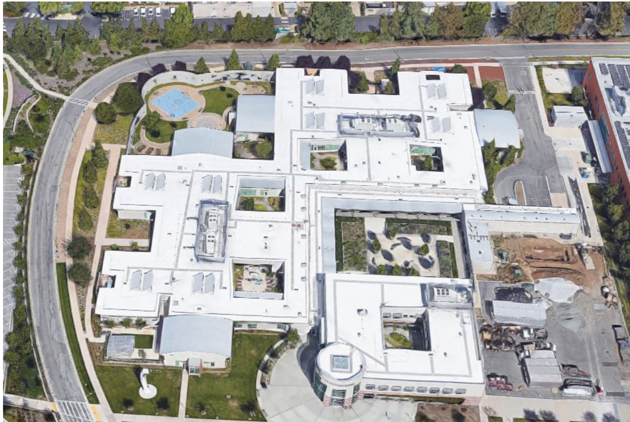
Figure 6.200 Aerial of VAMC Palo Alto
