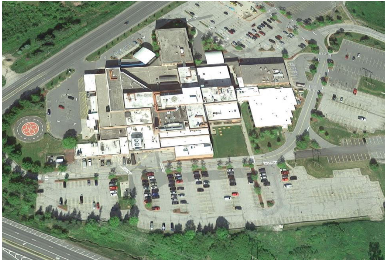
Figure 6.80 Aerial of Central Vermont Medical Center
