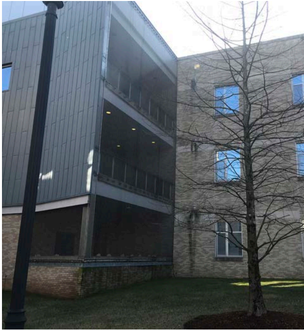
Figure 6.151 Essex County Hospital Center Porch, Reference Key Note #1
