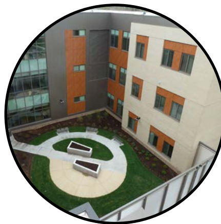
OUTDOOR ACTIVITY AREA Access to nature supports a therapeutic environment for both patients and staff. Outdoor areas shall be located and designed to prevent
