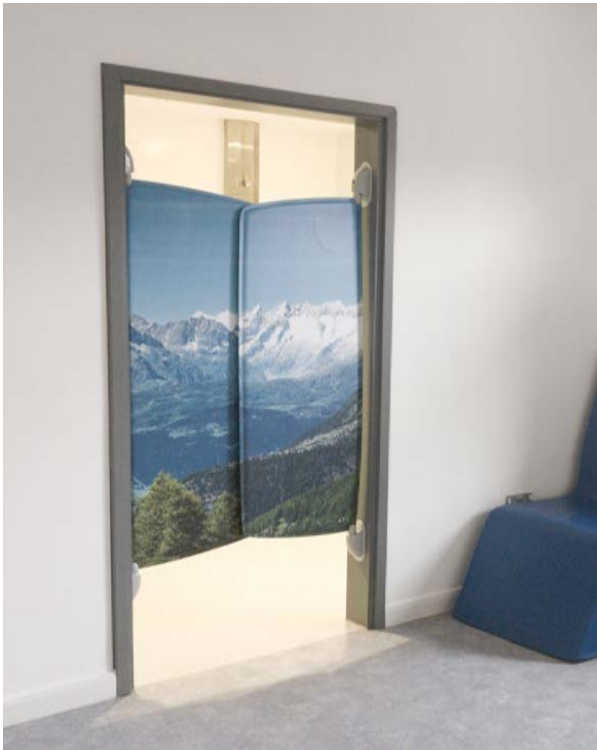
Figure 4.8 Example of IPMH soft suicide prevention toilet/shower room doors. Graphics applied to the door can enhance the inpatient room. Magnets, velcro or ant-ligature hinges are use for this application.
