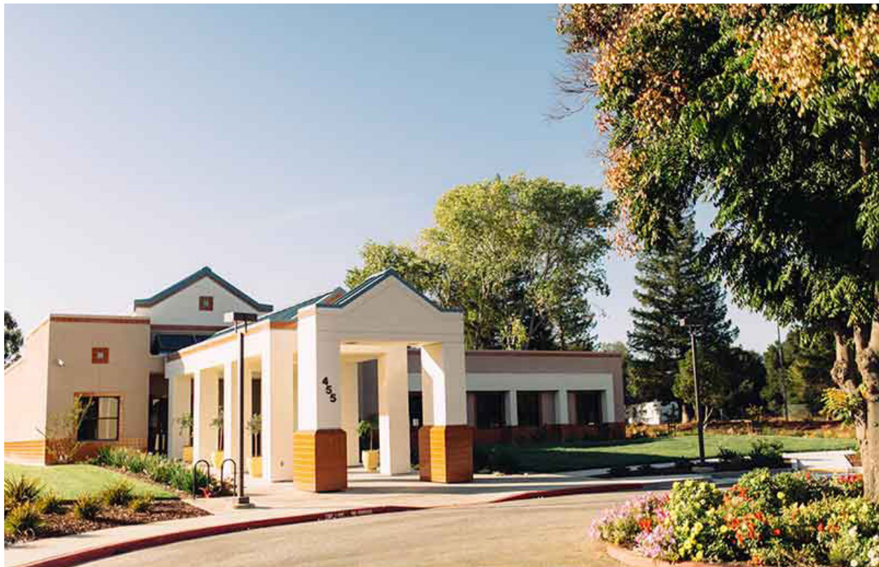
Figure 6.222 Main Entry of San Jose Behavioral Hospital
