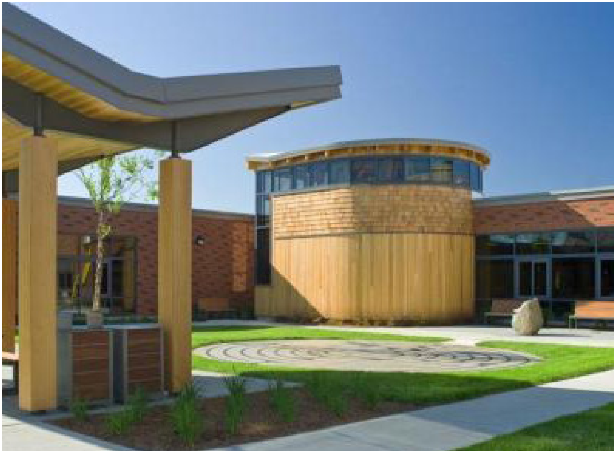
Figure 6.84 Main Courtyard of Vermont State Psychiatric Care Hospital
