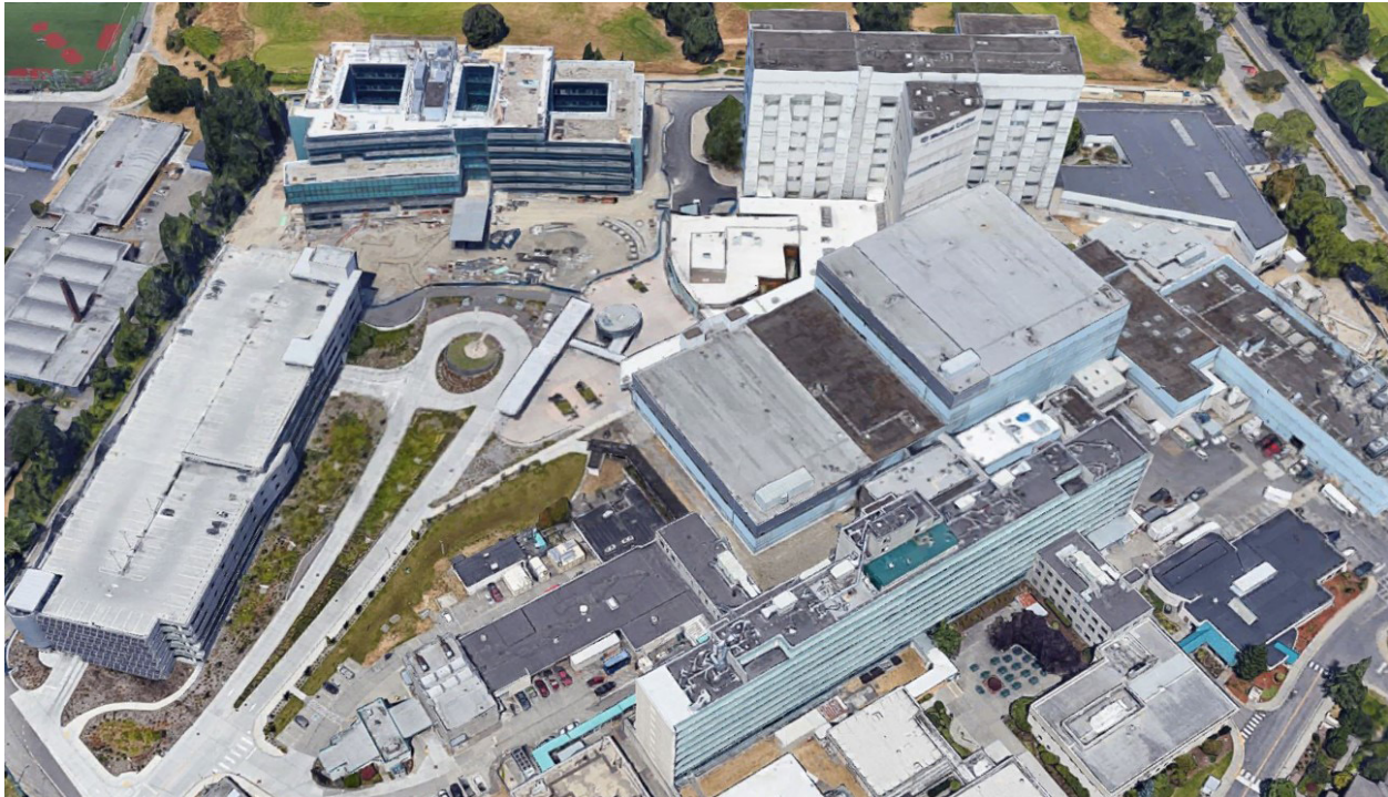
Figure 6.244 Aerial of VAMC Puget Sound
