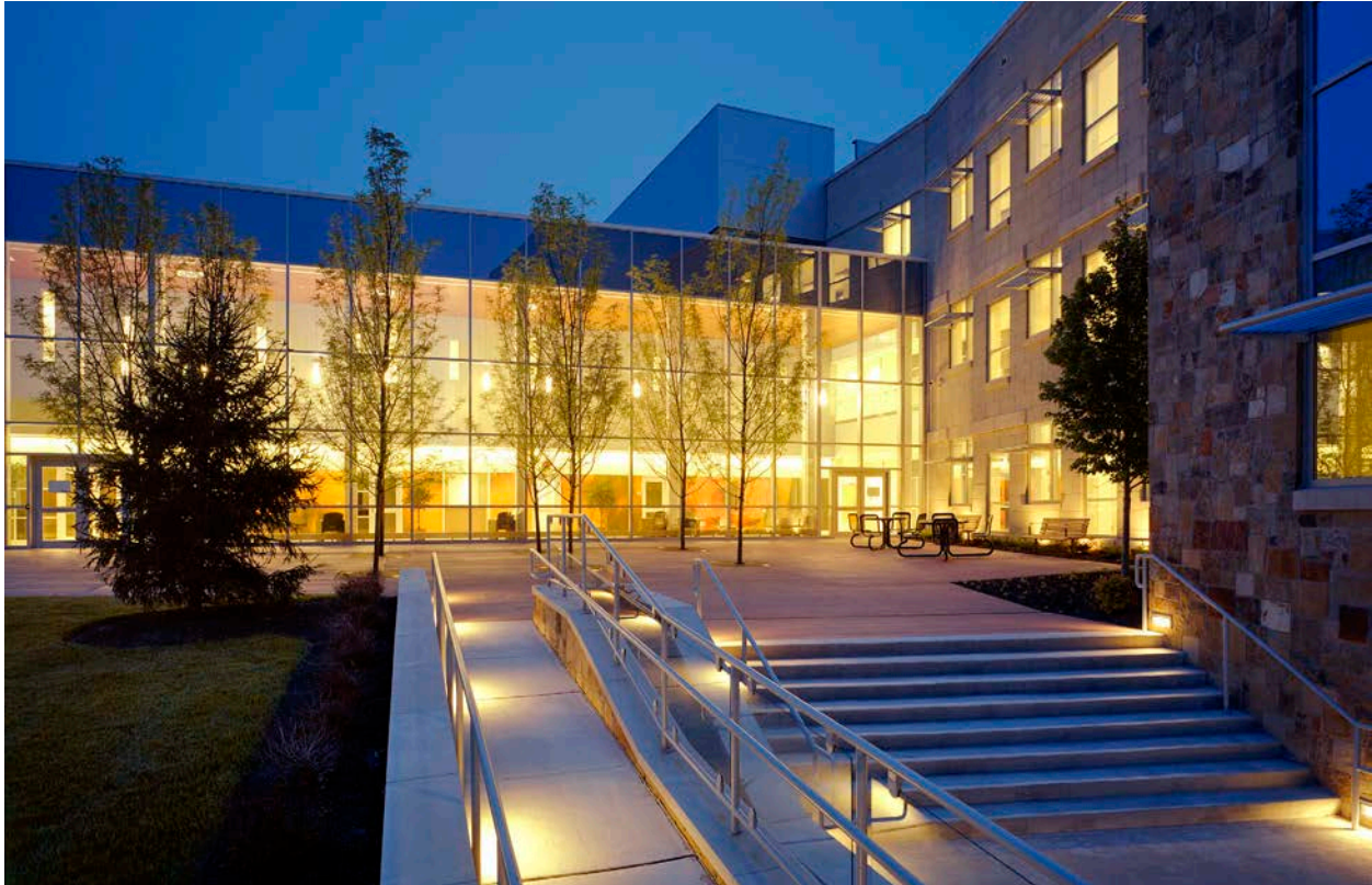
Figure 6.149 Courtyard of Essex County Hospital Center
