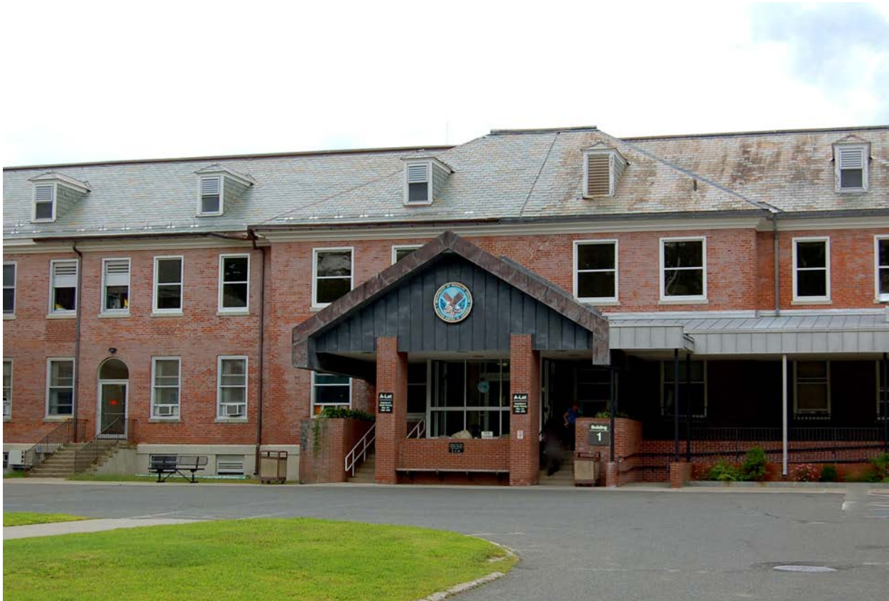
Figure 6.52 Main Entry of VA Central Western Mass.
