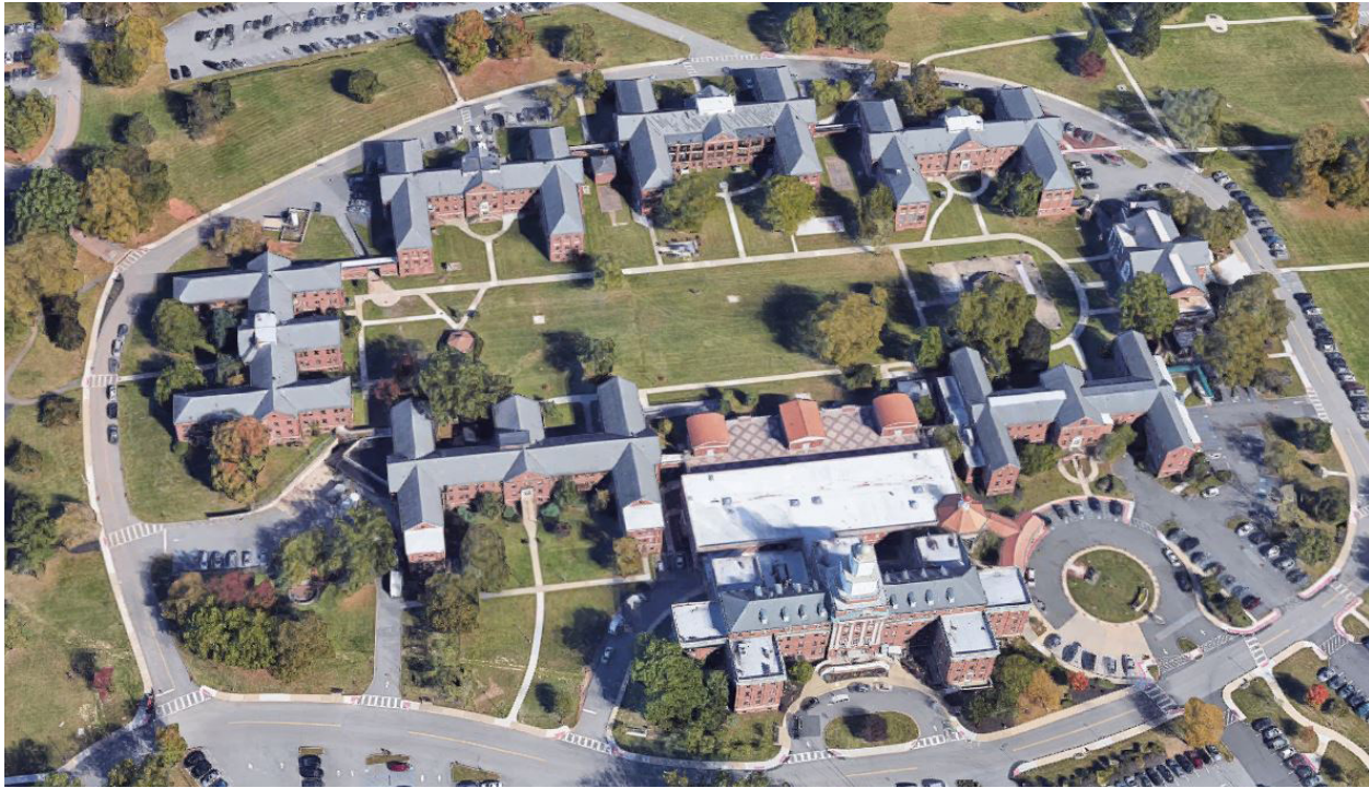
Figure 6.162 Aerial of VA Lyons + Domiciliary
