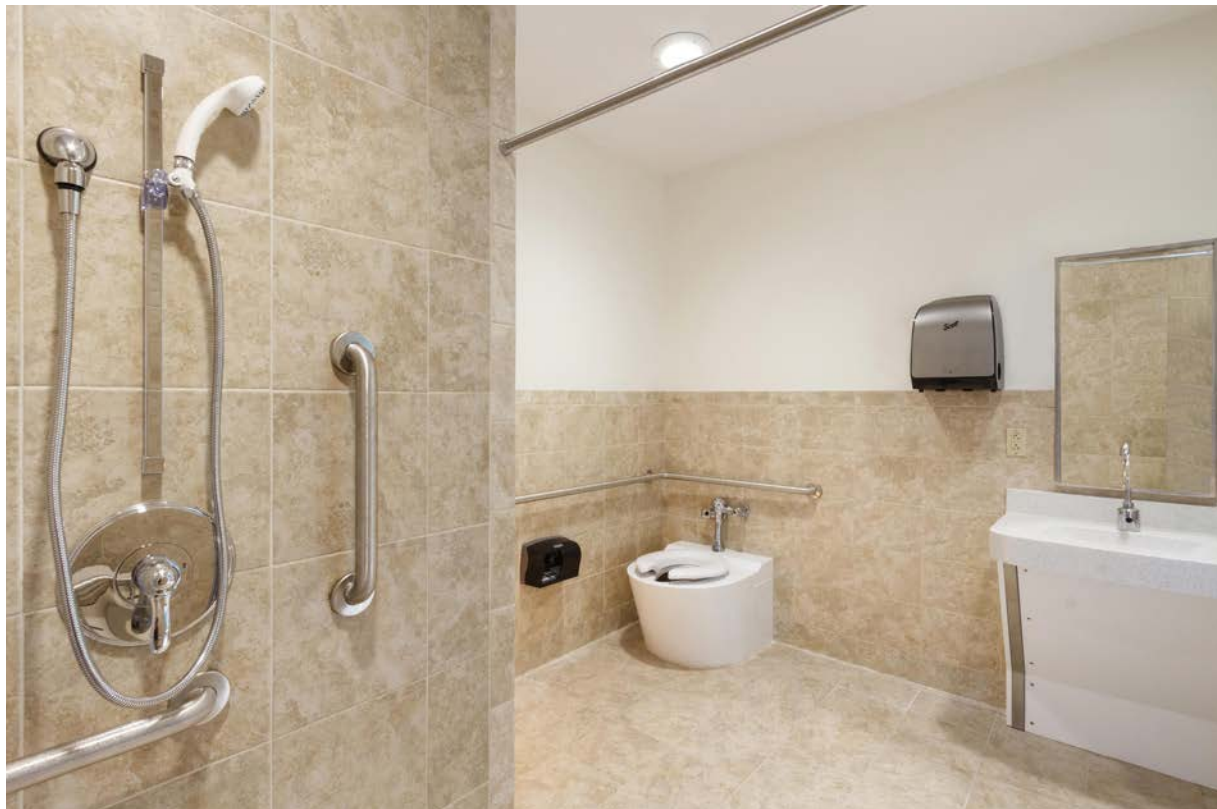
Figure 3.29 Providing a commercial grade fitting, fixtures and finishes for durability in the RRTP bathrooms doesn't require the use of anti-ligature devices. Source: West Palm Beach VAMC Domiciliary (AIA Architects + Planners, Inc.)
