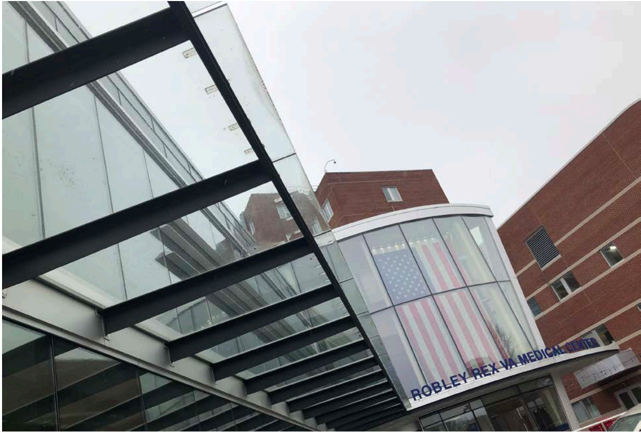
Figure 6.121 Main entrance of VAMC Louisville
