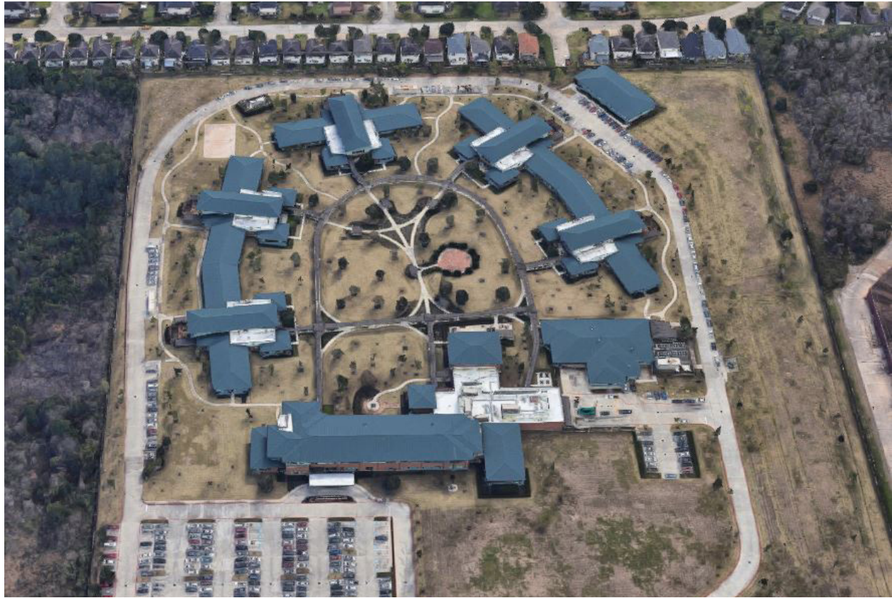
Figure 6.106 Aerial of Menninger Clinic, Houston, TX
