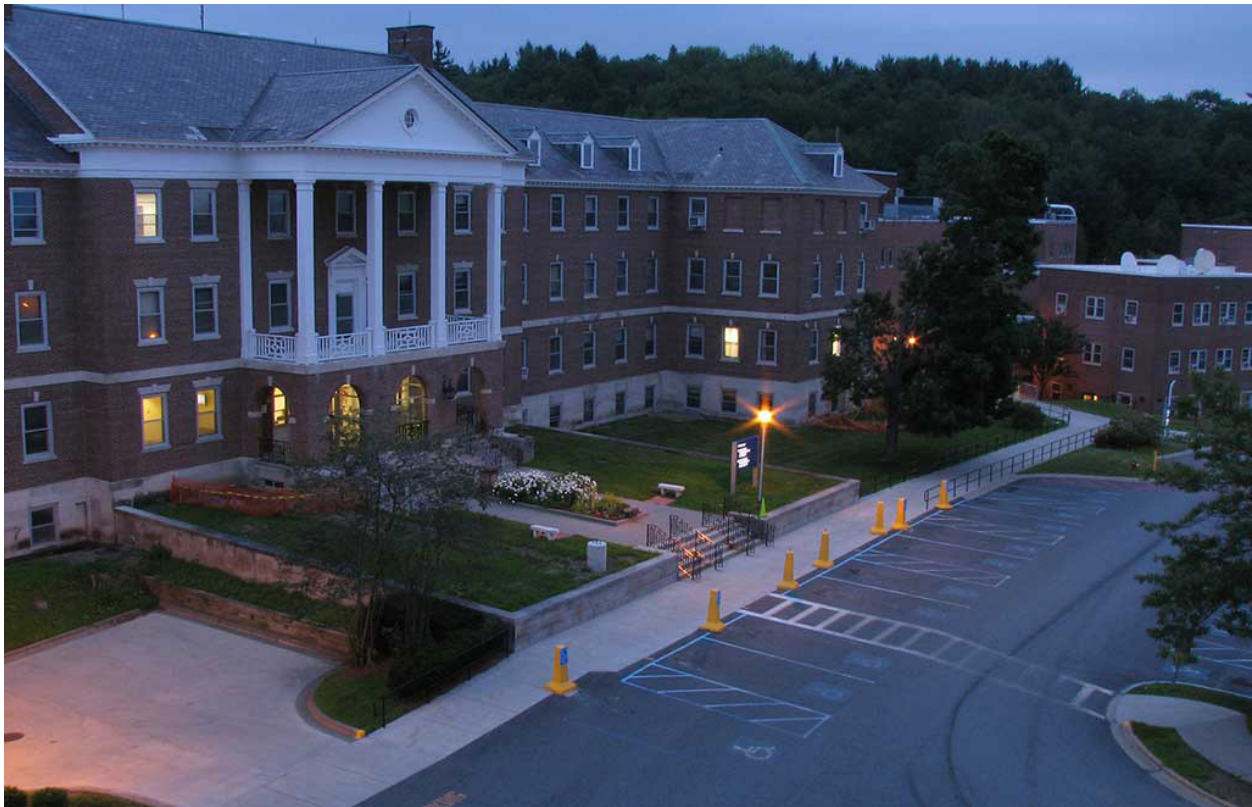
Figure 6.74 Main Entry of VAMC White River Junction
