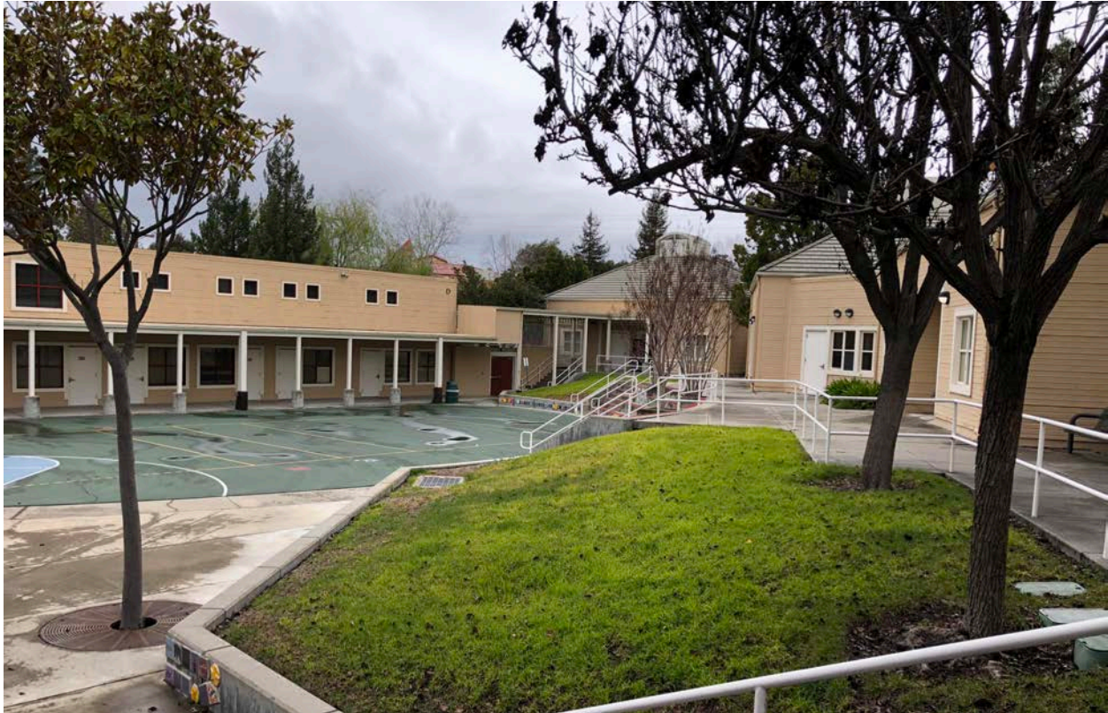
Figure 6.187 Main Courtyard of Willow Rock
