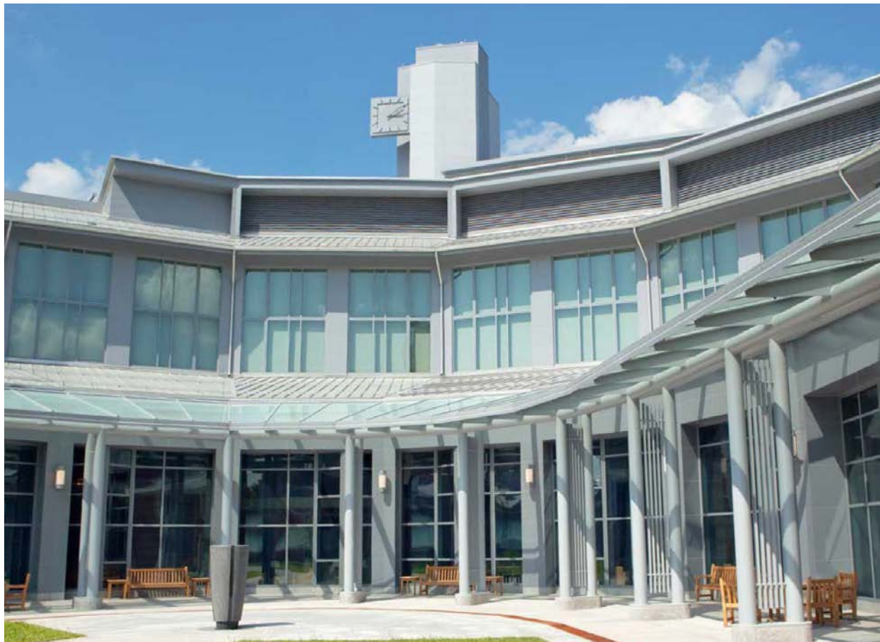
Figure 6.61 Interior of Worcester Adult Recovery Center & Hospital
