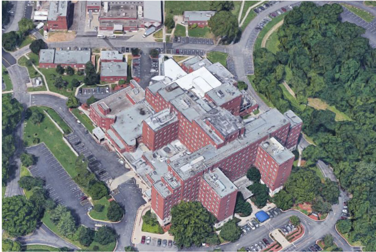
Figure 6.120 Aerial of VAMC Louisville, Louisville, KY
