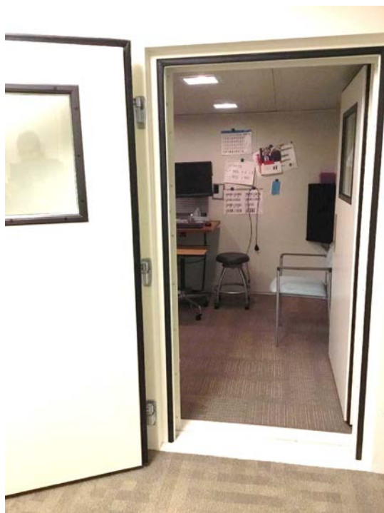
Figure 120: Booth Entrance – Flush Threshold
