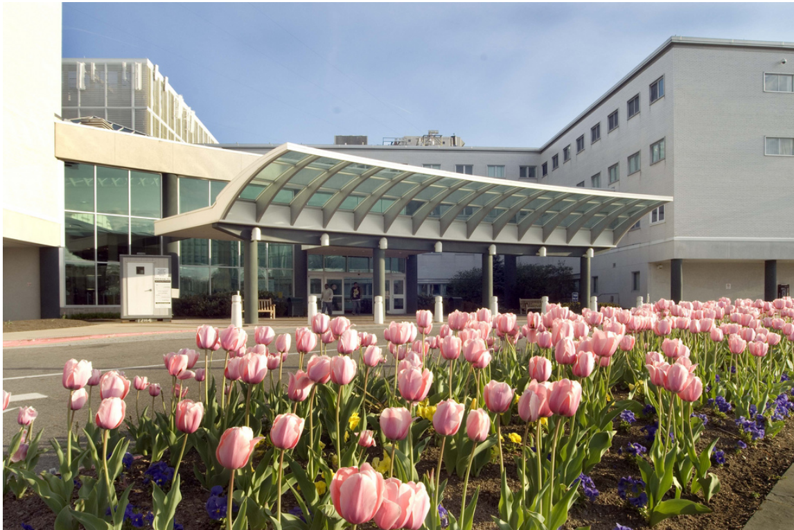
Figure 113: Washington, DC VAMC Main Entrance
