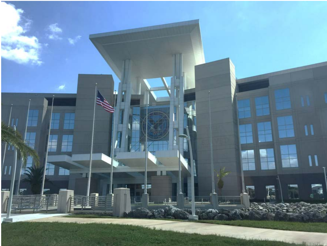
Figure 100: Orlando VAMC Main Entrance
