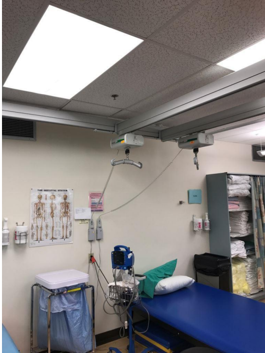
Figure 26 – two travelling rails at PT
