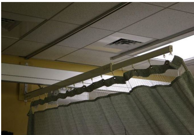
Figure 30 – telescoping privacy curtains extended
