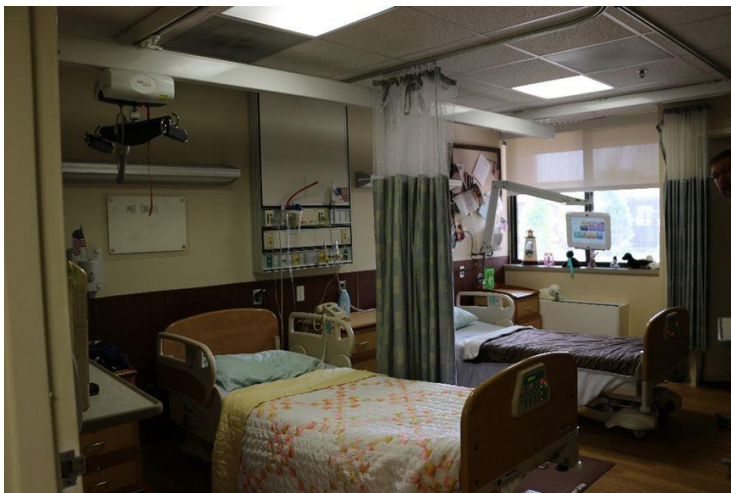
Figure 9 – conflict of travelling rail with privacy curtain
