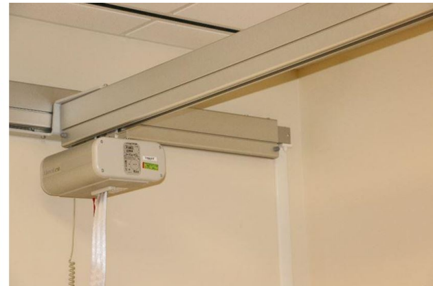
Figure 37 – wall mounted fixed rail parallel to wall
