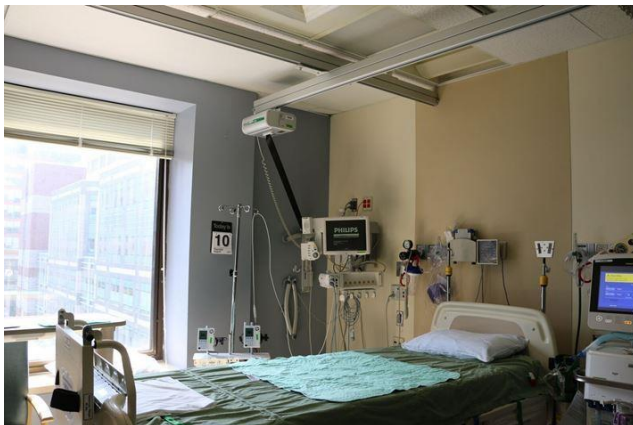
Figure 20 – travelling rail extending beyond fixed rail
