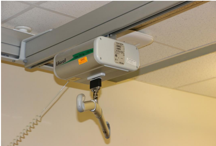
Figure 35 – end cap of travelling rail
