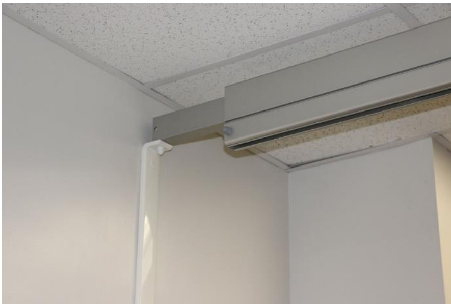
Figure 2-2 – wall-mounted end support of track
