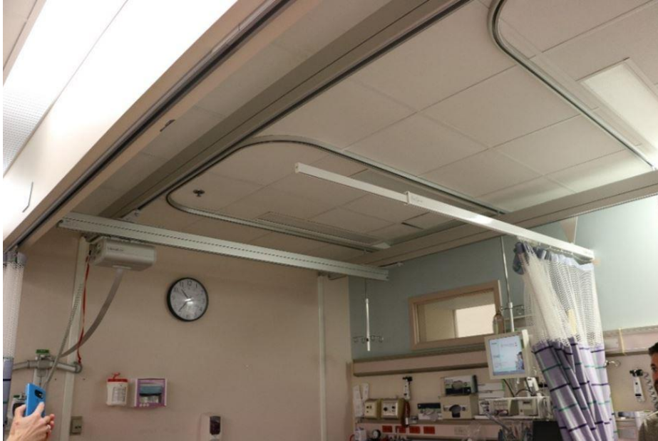
Figure 22 – PACU with telescoping privacy curtain
