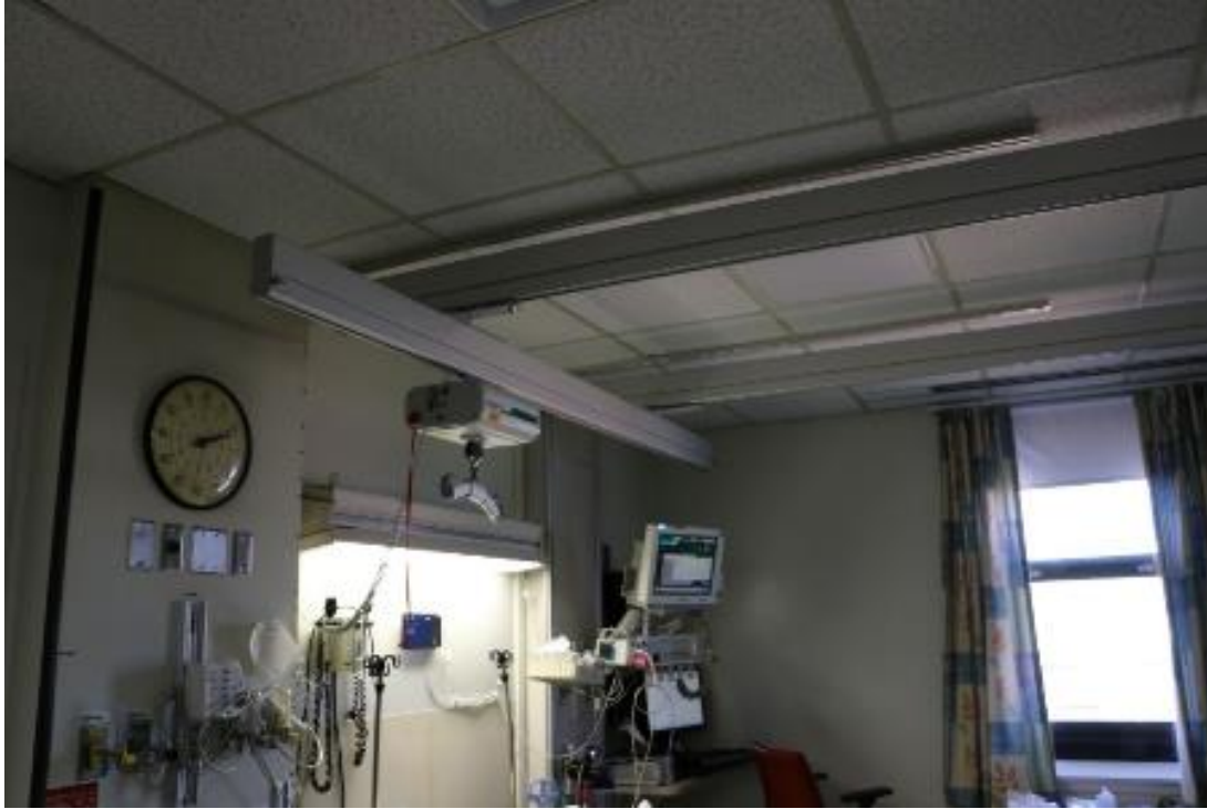
Figure 38 – lift with limited room access and coverage
