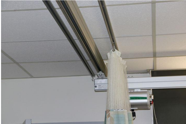
Figure 28 – lift/privacy curtain conflict
