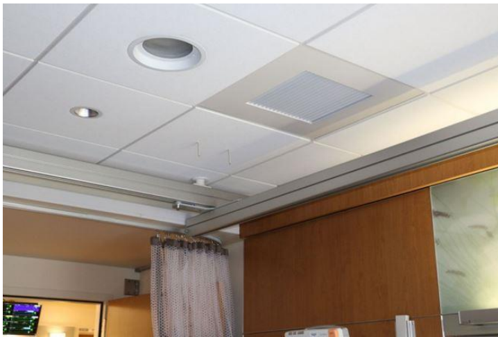
Figure 29 – privacy curtains outside lift access area in patient room
