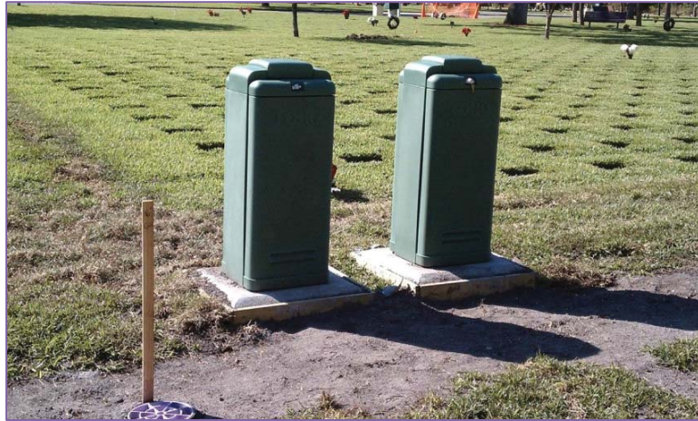
Photograph 2.05-4 Plastic Pedestal Controllers at Bay Pines National Cemetery
