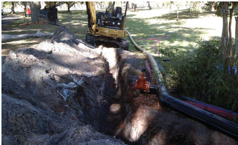
Photograph 2.05-1 HDPE Pipe Installation at Bay Pines National Cemetery
