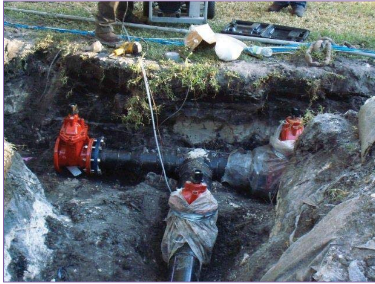
Photograph 2.05-2 Isolation Gate Valves on HDPE Pipe at Bay Pines National Cemetery
