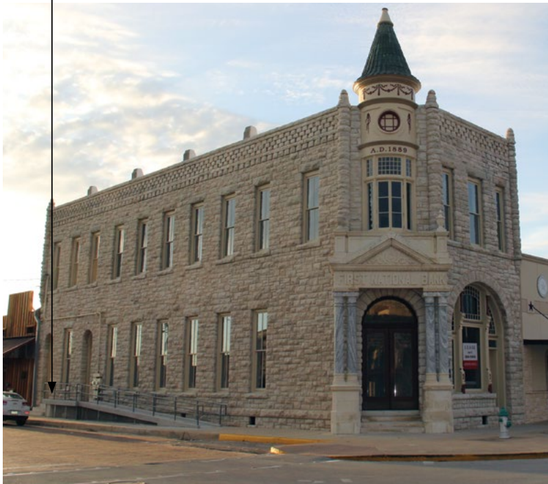
[53] This entrance ramp (right) is compatible with the historic character of this commercial building.
