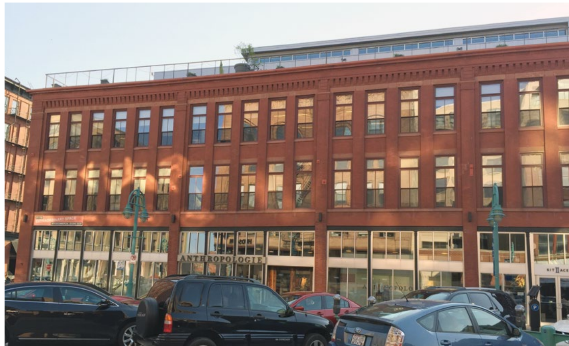
[64] Not Recommended: It is generally not appropriate to construct a rooftop addition on a low-rise, two- to three-story building such as this, because it negatively affects its historic character.
