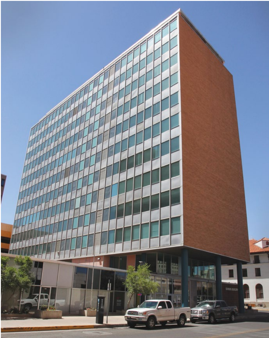
[30] Rather than replace the original curtain wall system of the 1954 Simms Building in Albuquerque, NM, with a different color tinted glass or coat it with a non-historic reflective film, the HVAC system was updated to improve energy efficiency. Photo: Harvey M. Kaplan.
