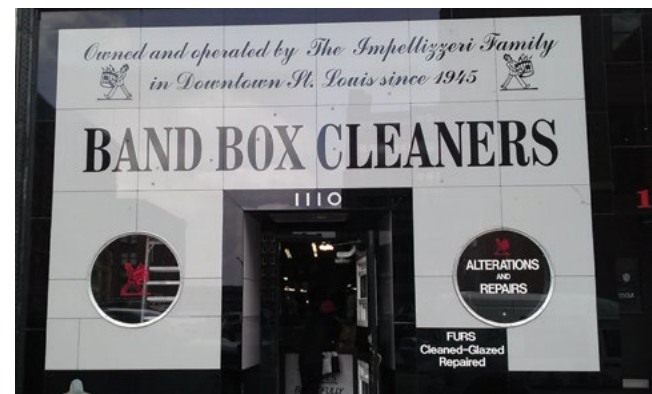
[14] The signage is an original and integral part of this historic Carrara glass storefront.
