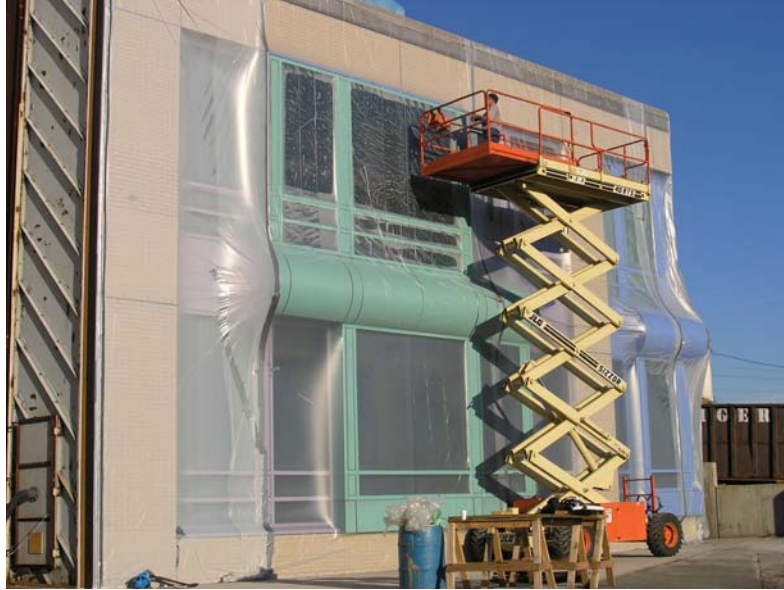
Figure 1. Lab mockup during ASTM E283 air infiltration test
