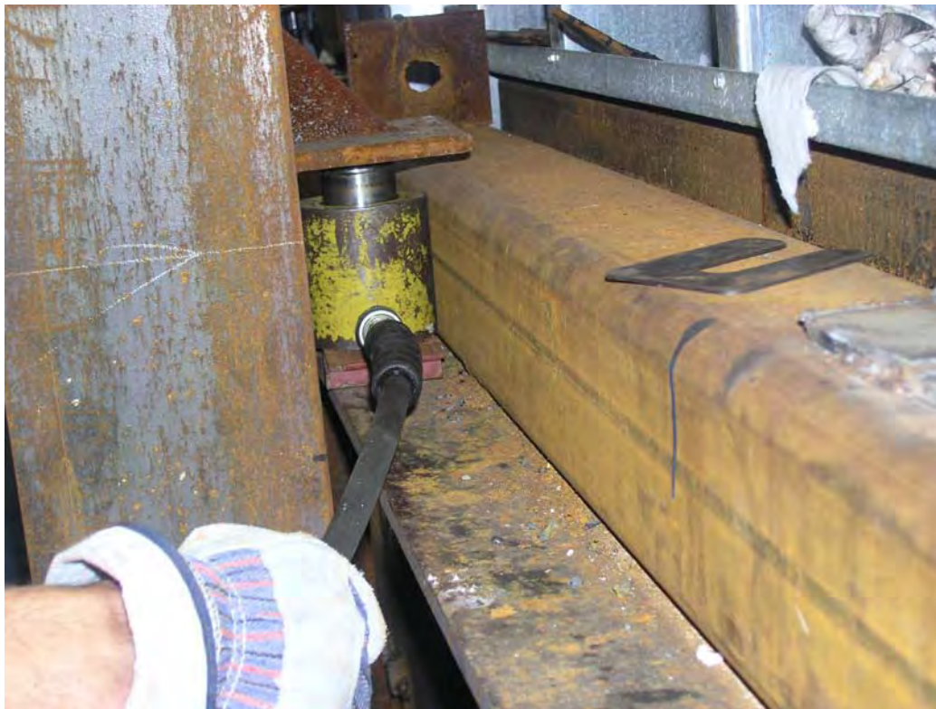
Figure 4 Installing hydraulic jacks to simulate inter-story drift.
