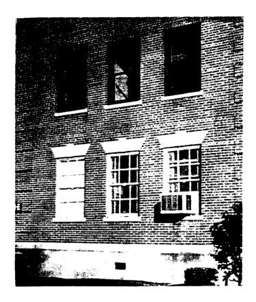
Figure 4-18. Historic Windows Inappropriately Replaced.
