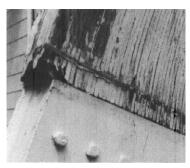
Figure 4-6. (C) Outward displacement evidenced by shear at the arch base.
