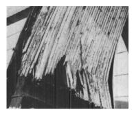
Figure 4-6. (D) Severe decay and failure of laminations.
