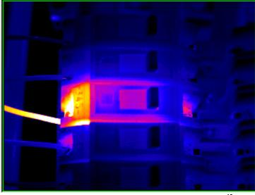
Figure B-9: Infrared Image of a 120 Volt Power Panel<sup>10</sup>
