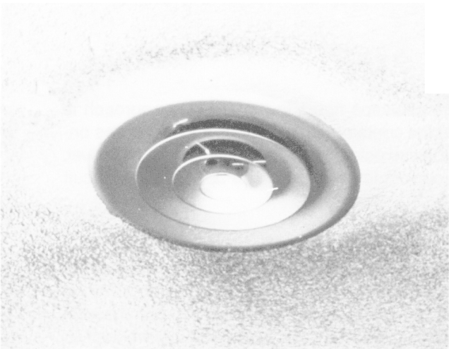
Airstream erosion from a heating vent
