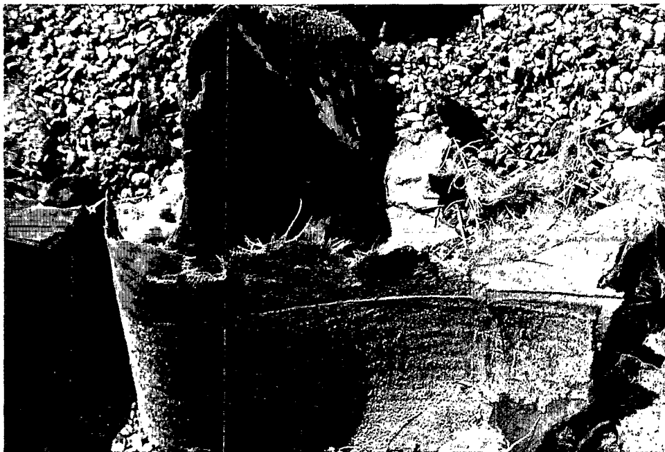
Figure 3. Asphalt roofing felts which are in poor condition. Notice the fibers protruding along the edge of this roofing felt.
