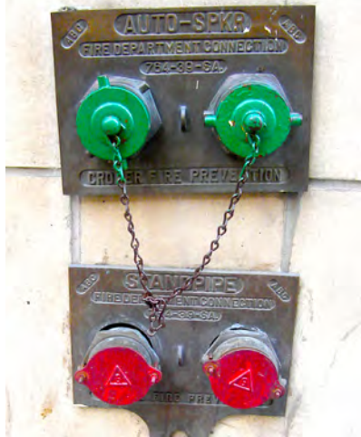
Figure 10.2. Separate sprinkler and standpipe FDCs. To feed both systems, at least one hose line must be connected to at least one inlet on each of the two FDCs.
