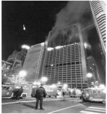
Figure 9.4. The Meridian Plaza high-rise fire.
