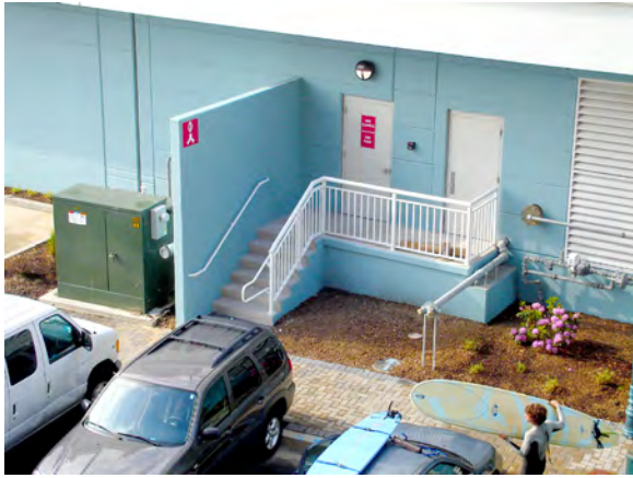
Figure 4.5. An outside door to a fire pump room identified by the red sign.
