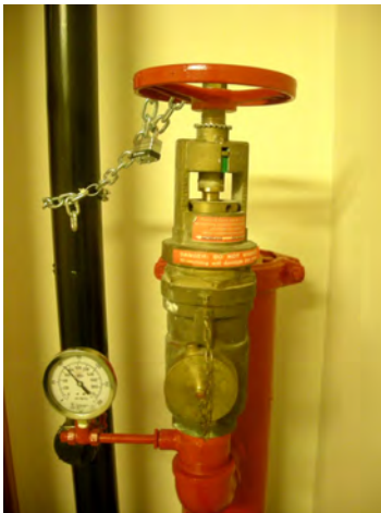
Figure 9.6. An FHC equipped with a pressure-regulating device.
