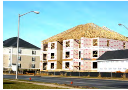
Figure 7.7. The building on the right is being constructed with wood trusses. The adjacent finished building shows no indication from the exterior that wood trusses were used in its construction.
