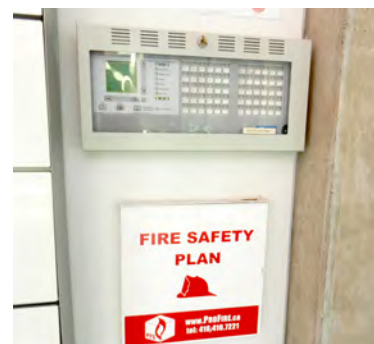
Figure 7.3. A cabinet containing building fire safety information for the fire service. The cabinet is conveniently located just below the fire alarm annunciator.
