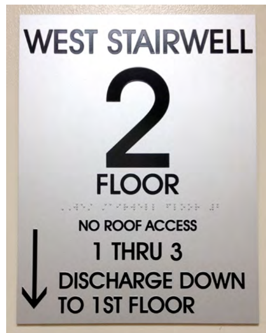
Figure 6.9. A stair identification sign.
