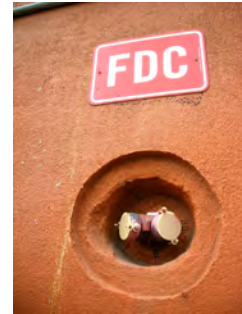
Figure 10.13. An FDC recessed into a wall. Note the notch on left prevents hose lines from kinking.
