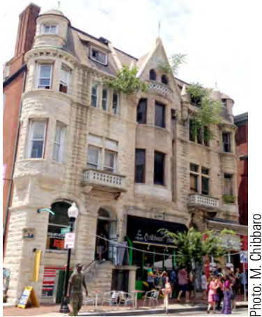
Figure 13.17. A building deteriorated to the point that trees are growing in it and major cracks are apparent.
