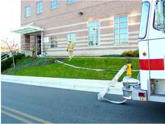
Figure 10.7. A fire hydrant in close proximity to an FDC (near the building entrance in the background). This allows the pumper to use its large-diameter intake hose to connect to the hydrant (foreground) and a pre-connected hose line to be stretched to the FDC (center of photo). Water will be supplied from the hydrant through the intake hose, through the pumper to boost pressure, and then through the hose line into the FDC.
