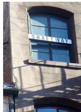
Figure 7.10. Exterior shaftway marking.
