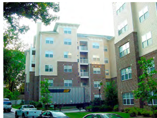
Figure 8.10. A building with six occupied levels from this vantage point. However, from a code standpoint, it is a four-story building because the top level is a loft and the bottom level is a basement mostly below grade. Its residential sprinkler system does not cover the combustible attic space or the truss spaces between floors.
