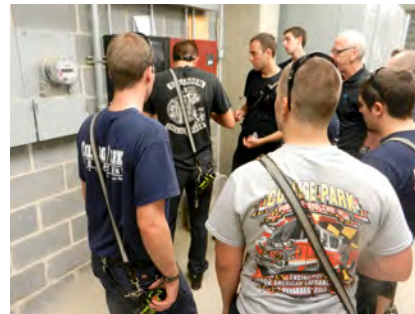
Figure 13.7. Building maintenance staff familiarizing firefighters with a fire alarm system in a new building.
