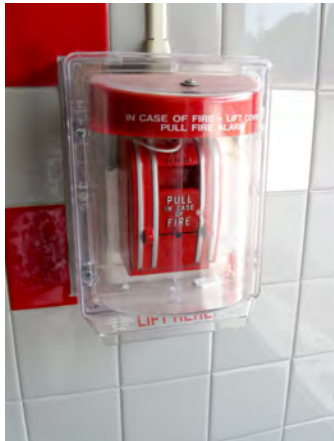
Figure 11.8. A manual pull station cover.
