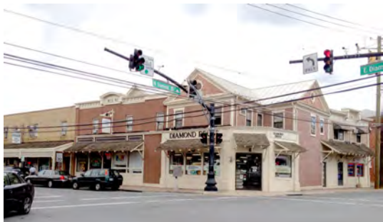
Figure 11.6. This building has multiple tenants with different addresses fronting on two streets. Strobes outside each exterior tenant entry door indicate the tenant where an alarm originates.
