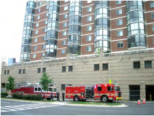
Figure 11.12. This high-rise building has three garage levels interconnected by open vehicle ramps. Those three levels have a single occupant notification zone.
