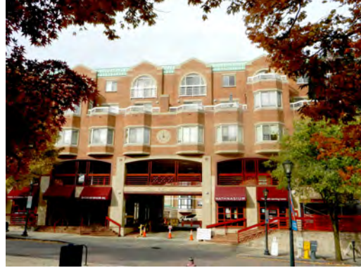
Figure 8.3. Some apartment units in this building span the fourth and fifth floors. Each two-story unit has a single entry door on the fourth floor.
