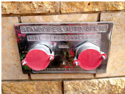
Figure 10.3. A combined sprinkler and standpipe FDC.
