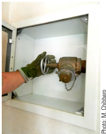
Figure 9.13. A FHC in a cabinet being checked by an inspector wearing a firefighting glove.
