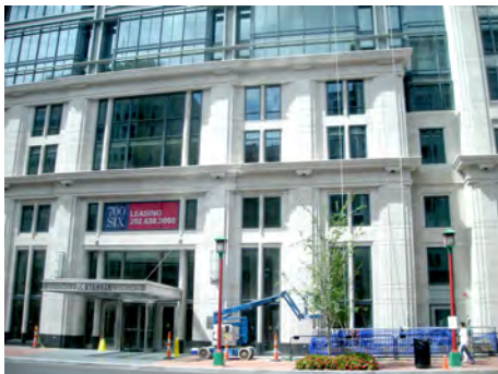
Figure 13.2. A new, partially-occupied, speculative office building.
