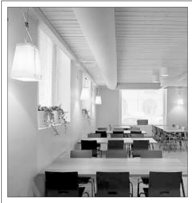
Half-round textile ducts in the Carlsson company's dining room (in Sweden) retain their shape even when not inflated with supply air.
