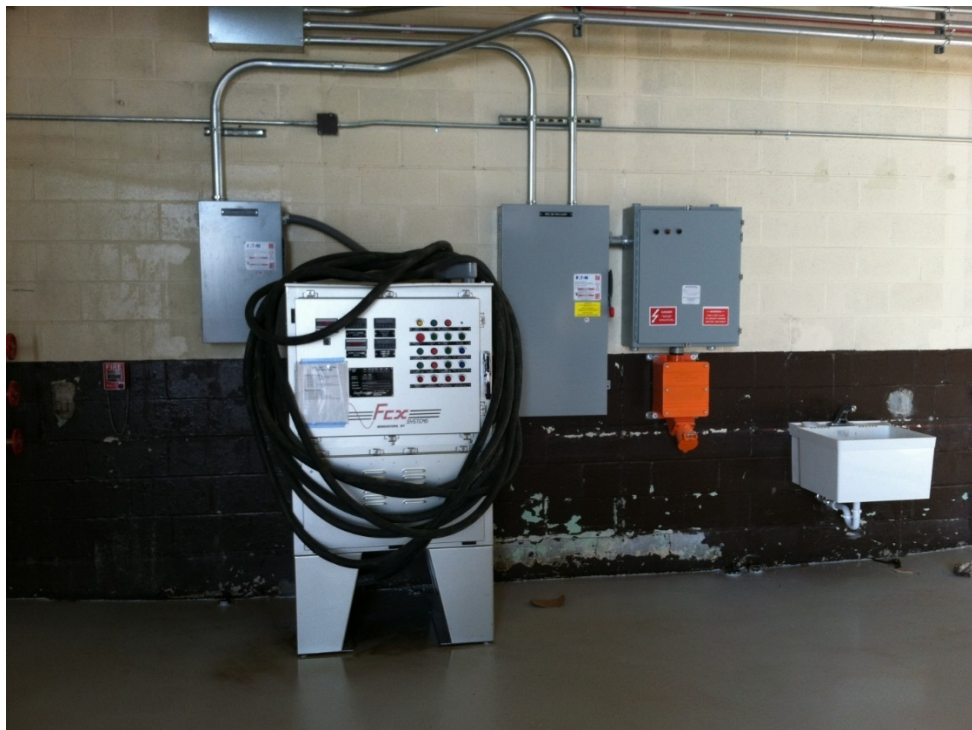
Figure E-16: Permanent Pedestals with 400 Hz, 120V, Communications and Compressed Air
