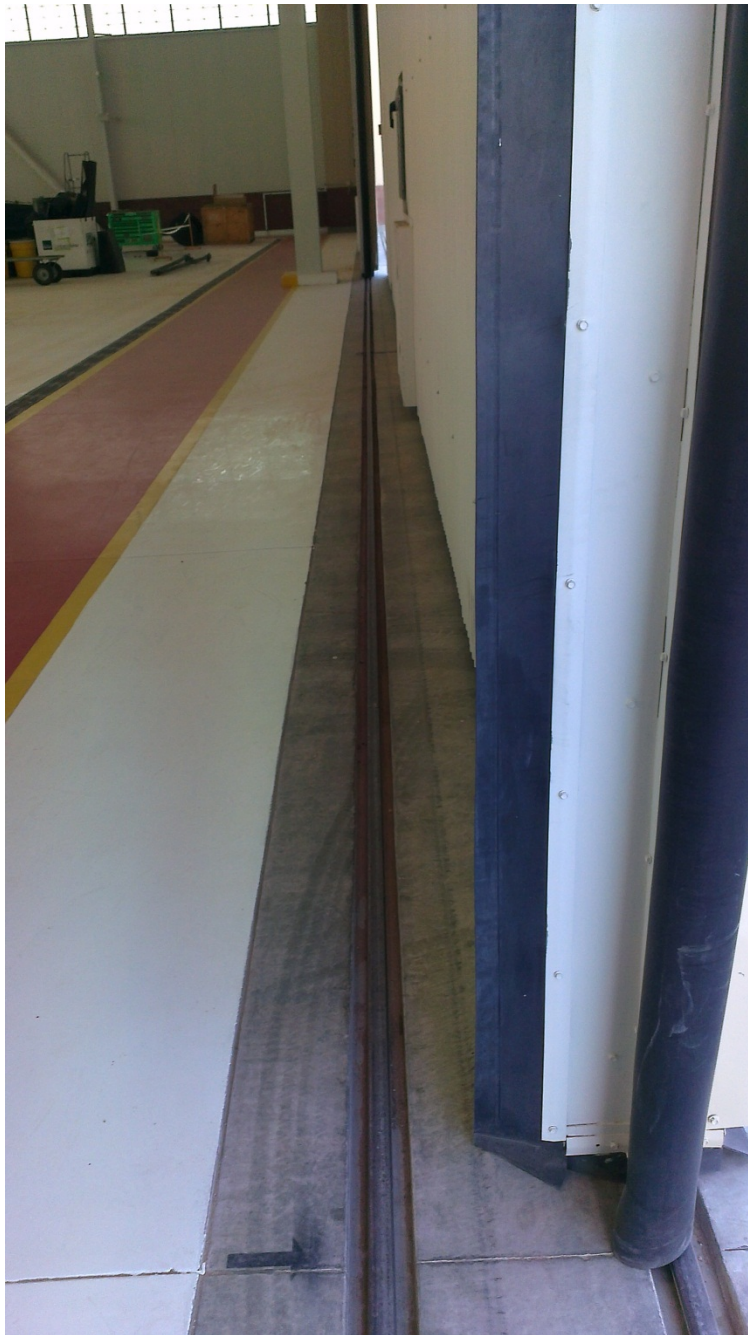
Figure E-12: Sliding Hangar Door Tracks
