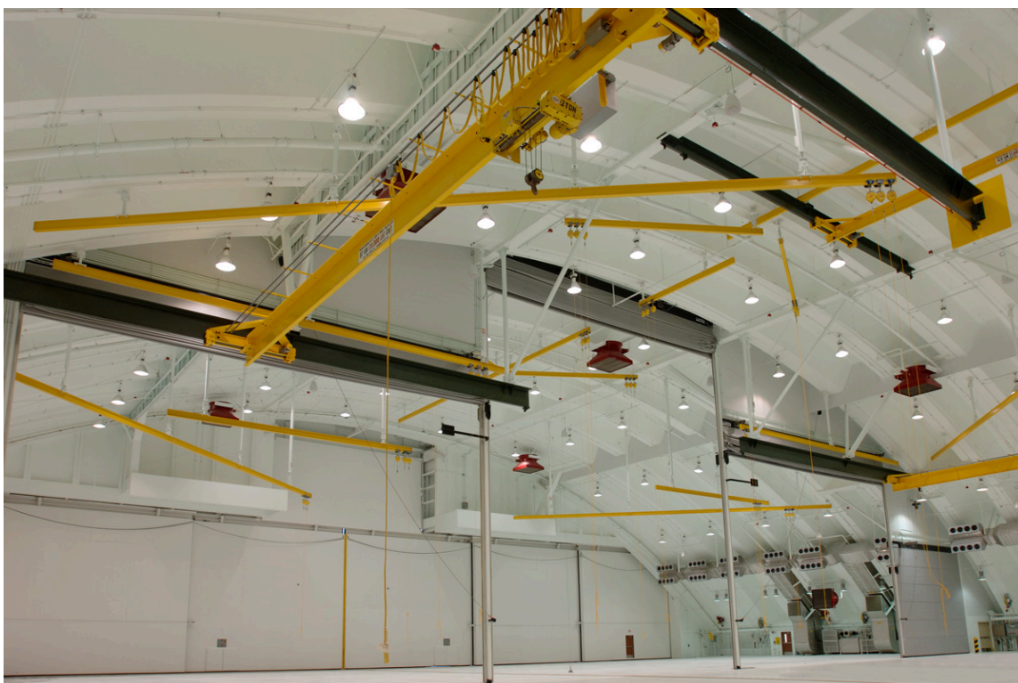
Figure E-10: Hangar Bay with Bridge Cranes and Fall Arrest
