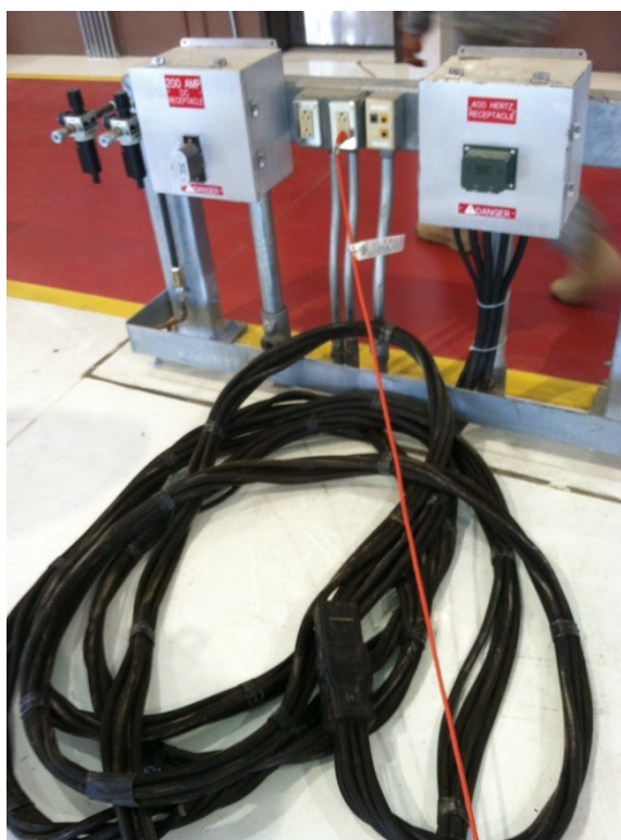
Figure E-16: Permanent Pedestals with 400 Hz, 120V, Communications and Compressed Air
