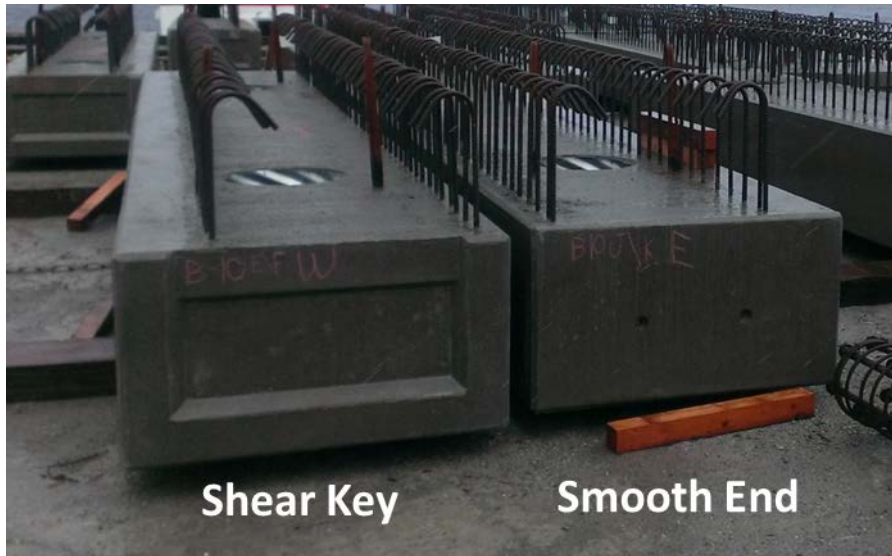
Precast Pile Cap Showing End Configurations
