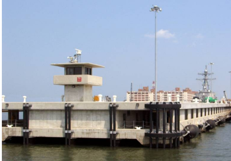
Figure 5-3 Guard Tower on Pier
