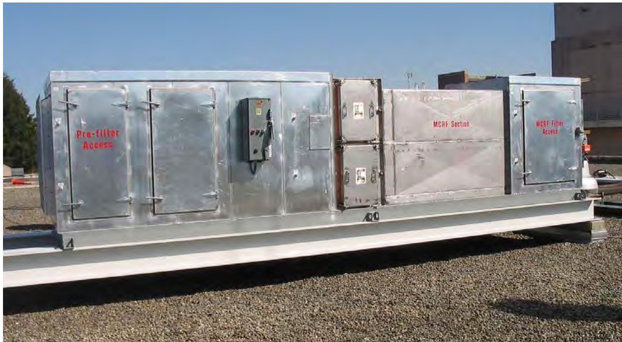
Figure G-12. Multi-Cell Radial-Flow (MCRF) Filtration Unit
