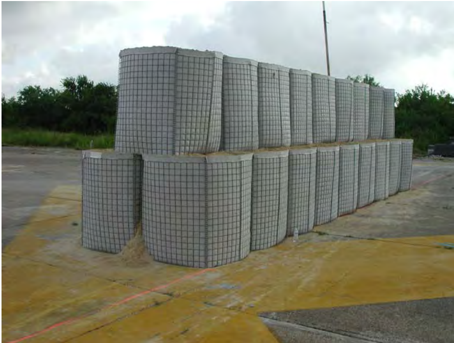
Figure E-3 Hesco Bastion Concertainer Barrier, Oblique View
