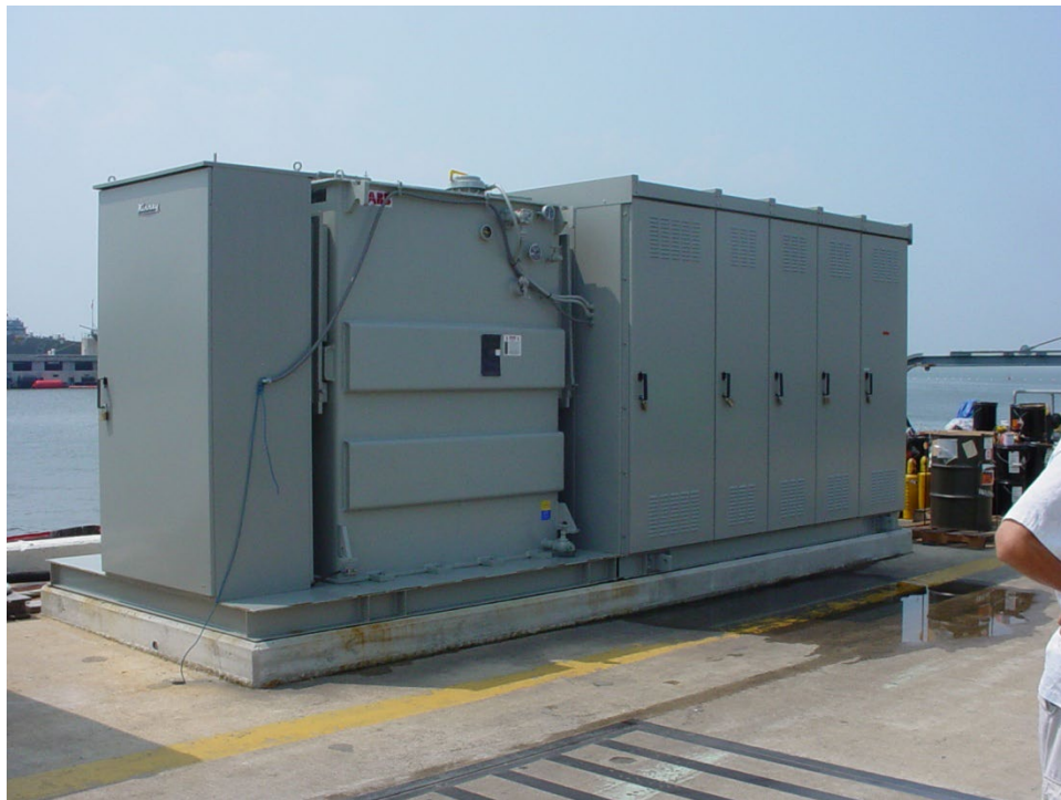
Figure 12-5. Skid-Mounted Substation with Single-Pole Connections
