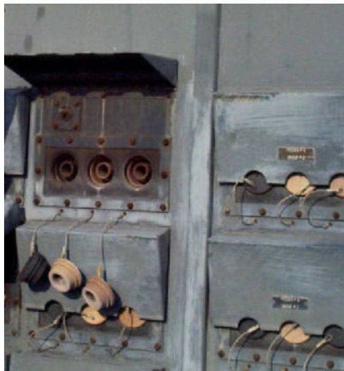
Figure 12-5. Skid-Mounted Substation with Single-Pole Connections
