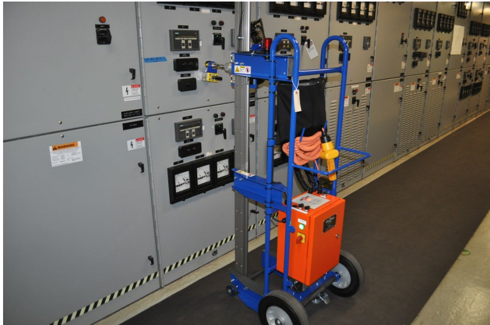
Figure 1. Remote Racking Mechanism
