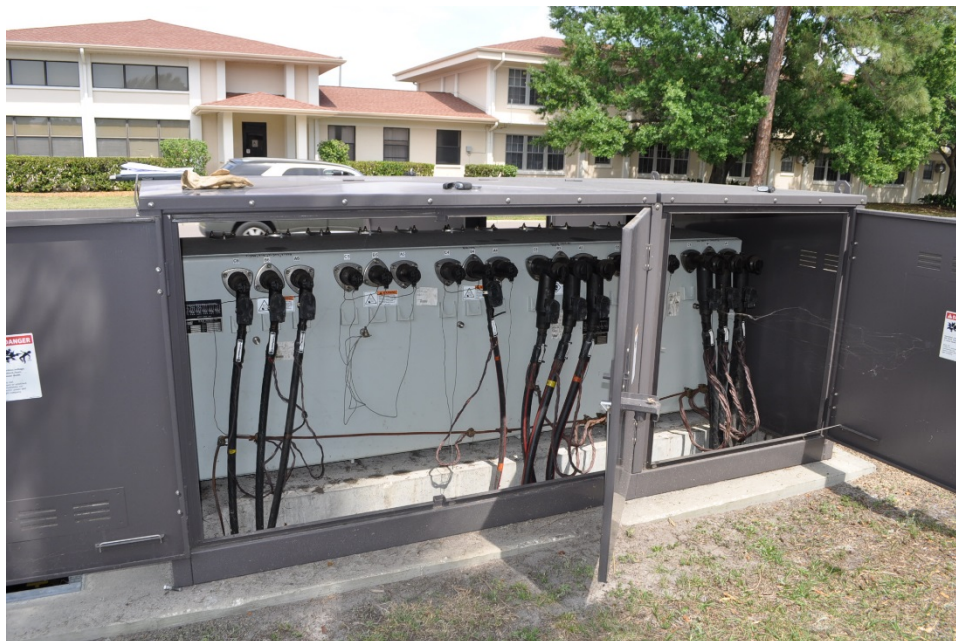
Figure D-2 G&W VFI Switchgear
