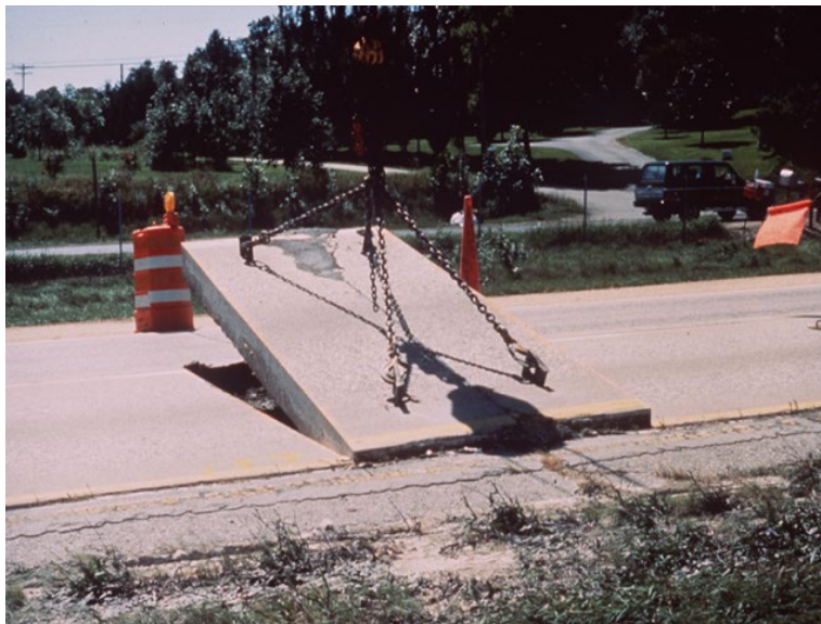
Figure 14-7 Lift-out Method
