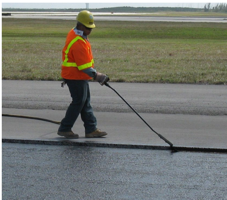
Figure 3-5 Hand-spraying Edge of Cut
