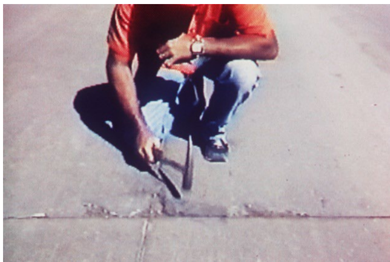
Figure 13-3 Sounding with a Hammer
