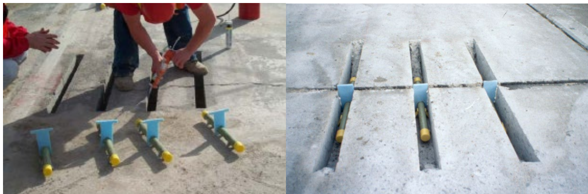
Figure 18-6 Use of Compressible Insert
