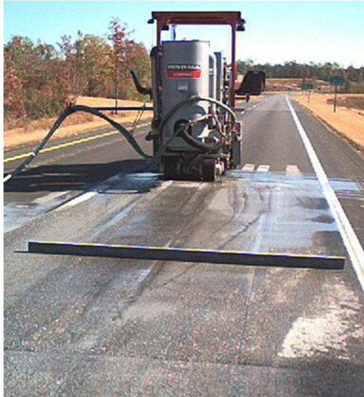
Figure 11-1 Diamond Grinding Equipment
