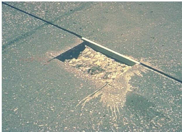
Figure 13-8 Compressible Insert
