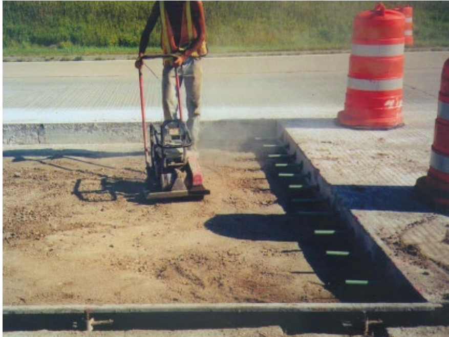
Figure 14-9 Patch Area Compaction
