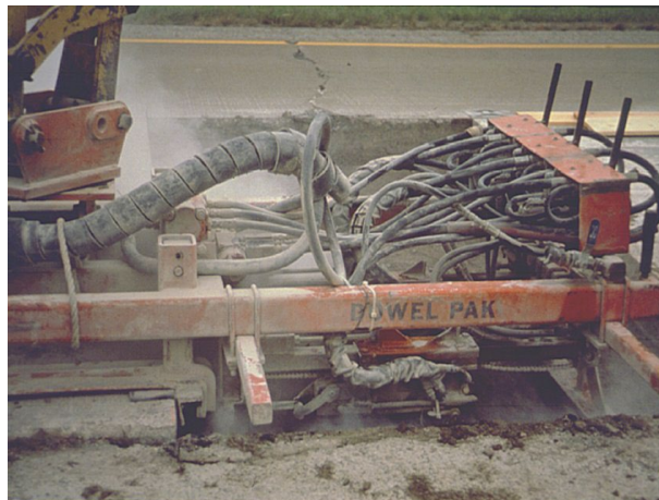
Figure 14-10 Drilling Multiple Holes at Mid-depth for Dowel Bars
