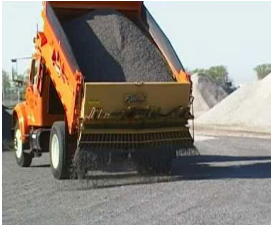
Figure 6-2 Applying Aggregate with Self-Propelled Hopper-type Spreader
