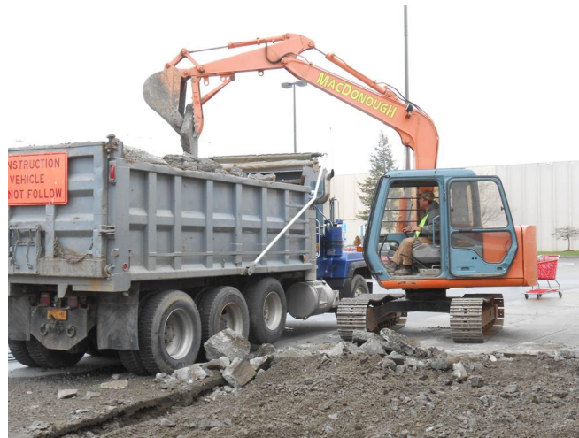
Figure 14-5 Concrete Removal Using Backhoe
