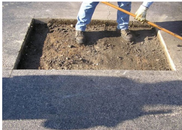
Figure 3-3 Damaged Pavement Removed by Sawing
