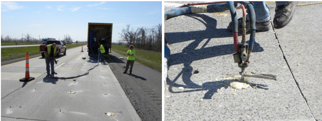
Figure 16-1 Polymer Subsealing Process
