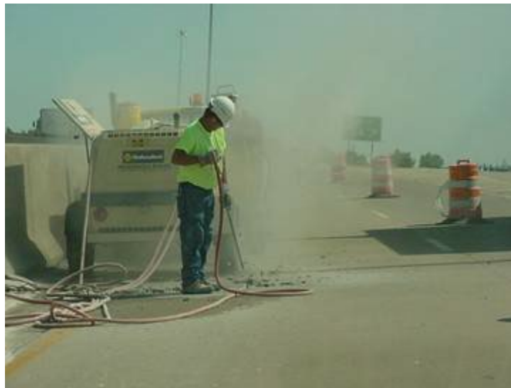
Figure 13-7 Cleaning Repair Area (Sandblasting/Water Blasting, and Air Blowing)
