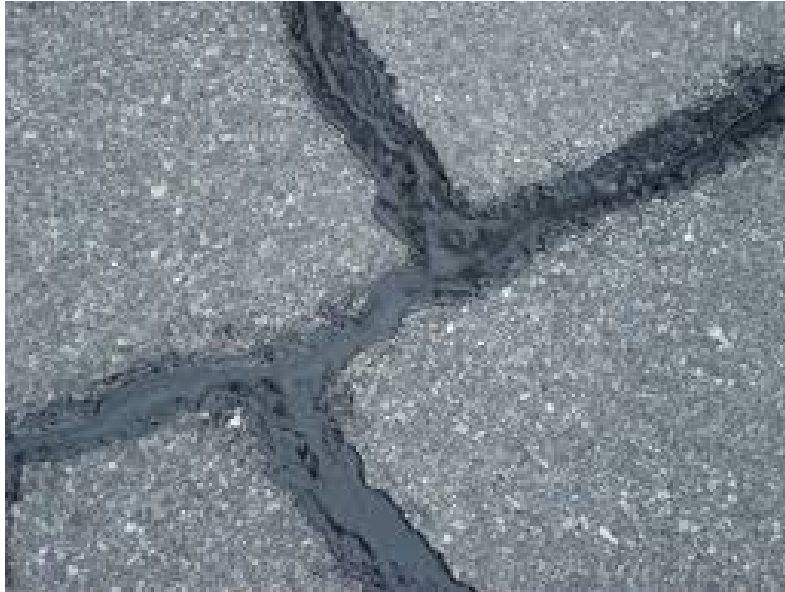
Figure 9-12 Crack After Sealing
