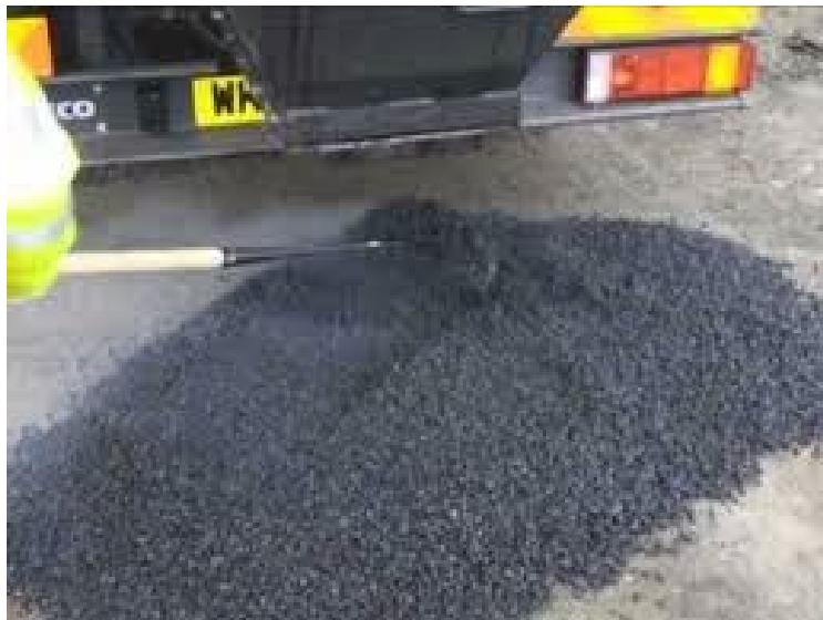
Figure 3-6 Overfill Prior to Compaction
