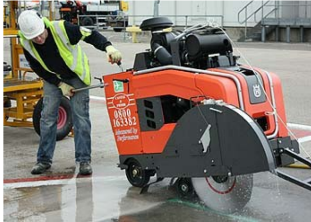
Figure 14-3 Diamond Blade Sawing
