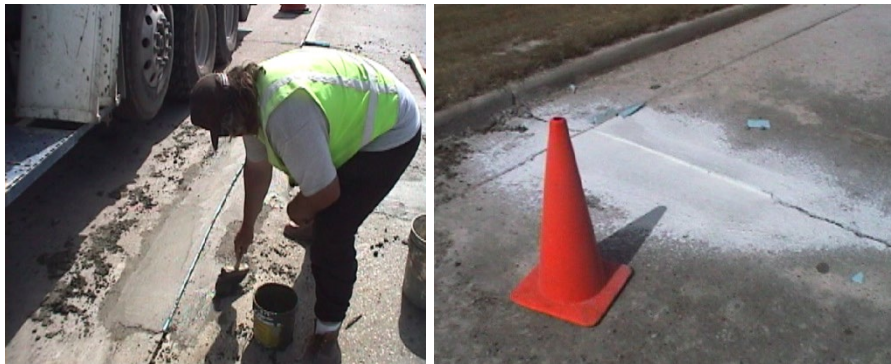
Figure 13-10 Finished Patches
