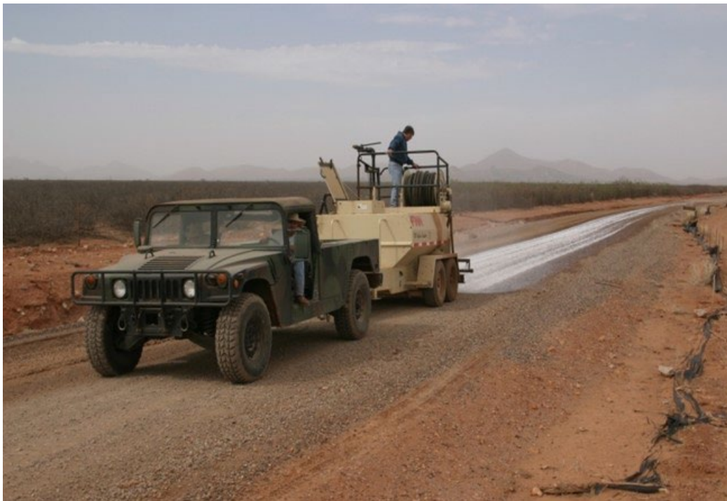
Figure 5-4 Applying Final Spray to Seal Road Surface After Compaction
