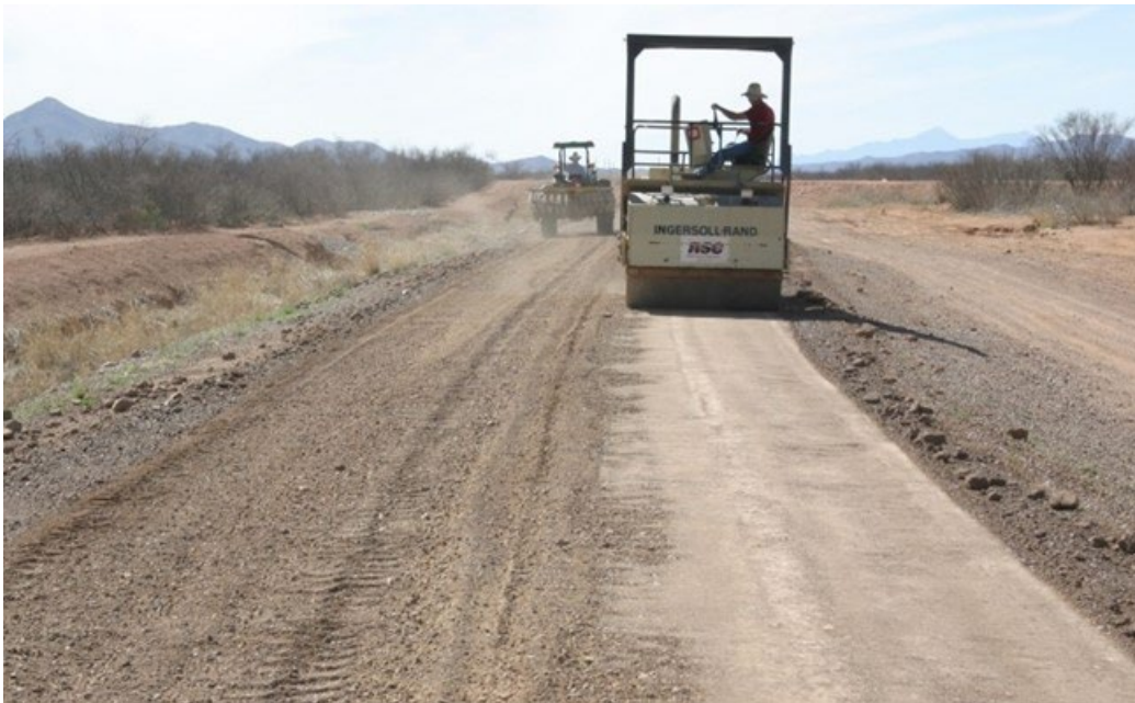
Figure 5-3 Compacting Road Surface After Mixing
