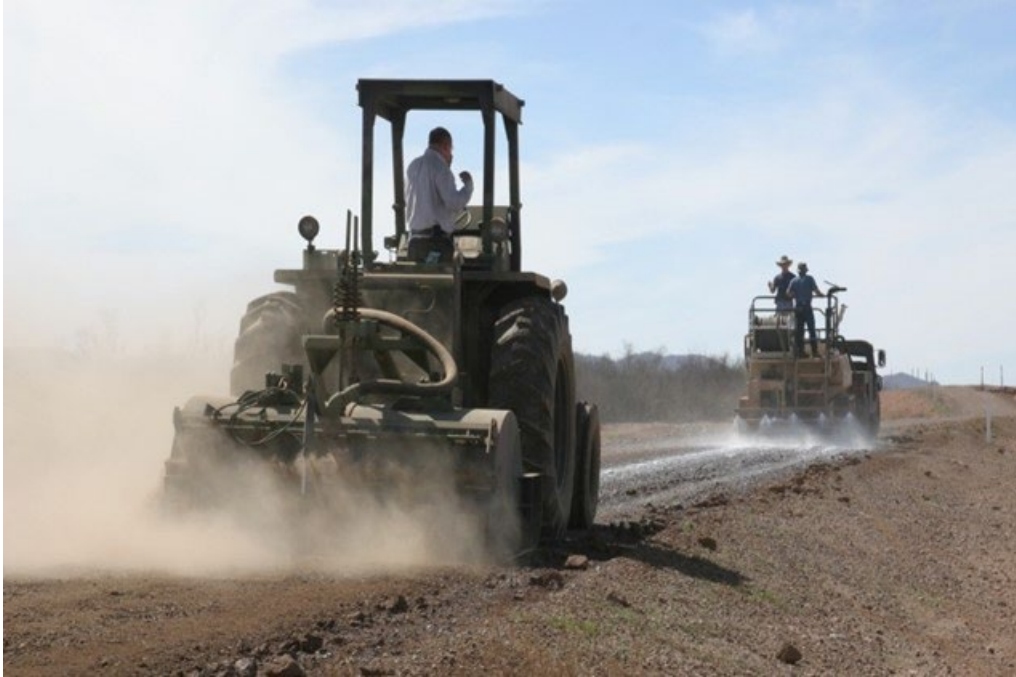
Figure 5-2 Applying Product with Hydroseeder and Mixing into Road Surface with Rotary Mixer
