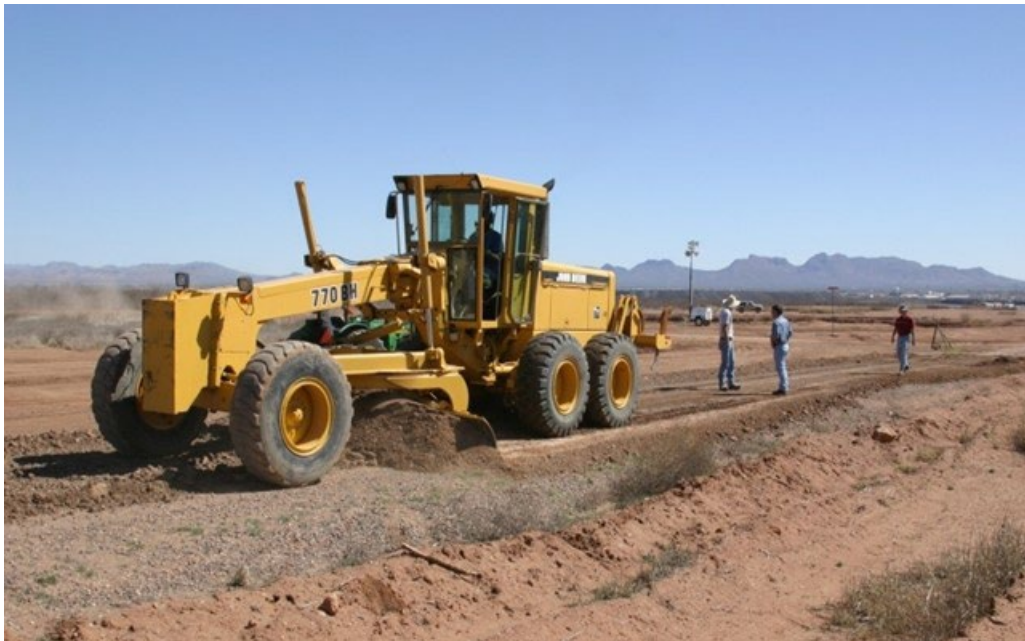
Figure 5-1 Grading Road Surface Prior to Treatment
