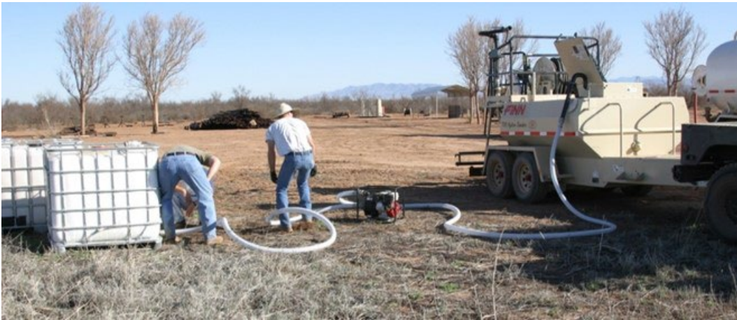
Figure 5-5 Filling Hydroseeder from Material Tote
