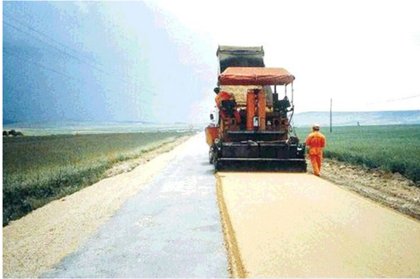
Figure 4-12 Granular Material Added to Achieve Compacted Thickness*
