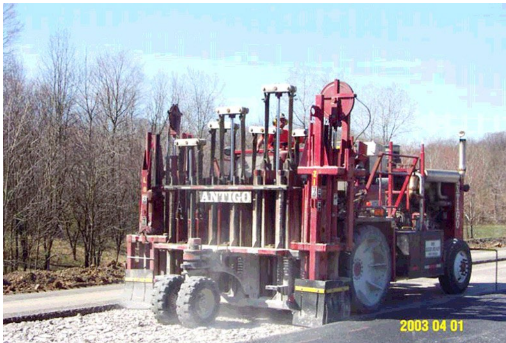
Figure 6-8 Rubblization Using MHB*
