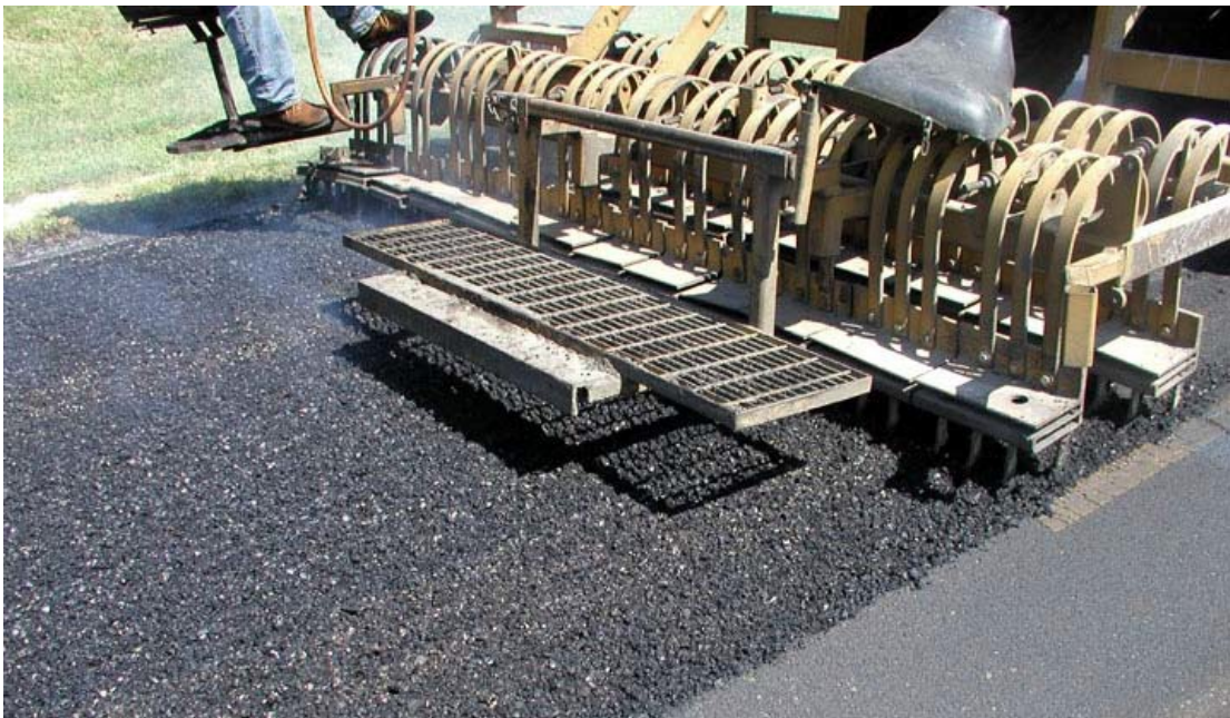
Figure 5-8 Surface Recycling Scarification Teeth*
