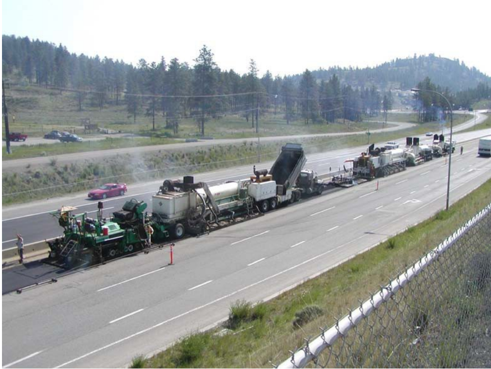
Figure 5-11 Example of Single Stage Remixing Train
