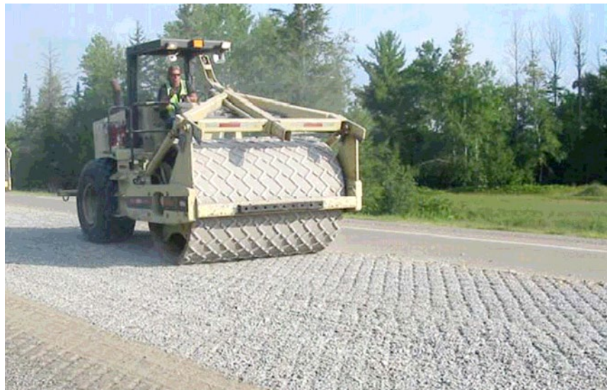
Figure 6-9 Z-Grid Roller Used on MHB Rubblized Pavement*
