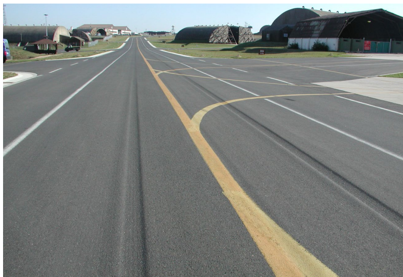
Figure 3-9 Rutting in the HMA Layers
