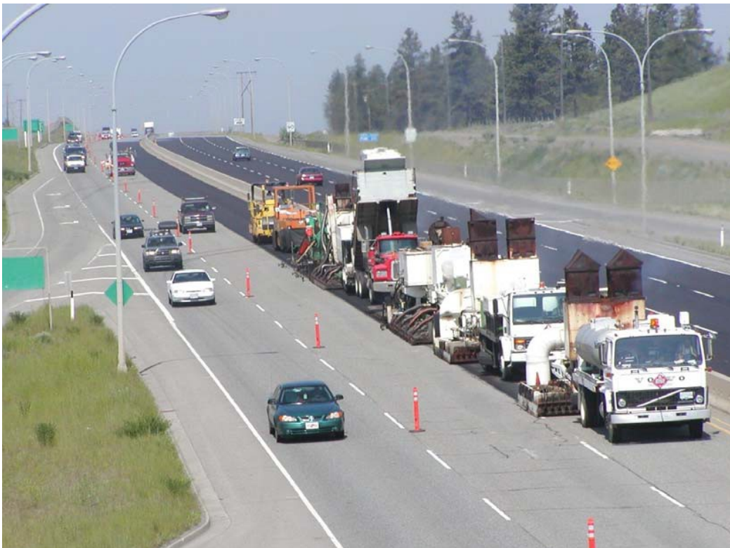
Figure 5-11 Example of Single Stage Remixing Train
