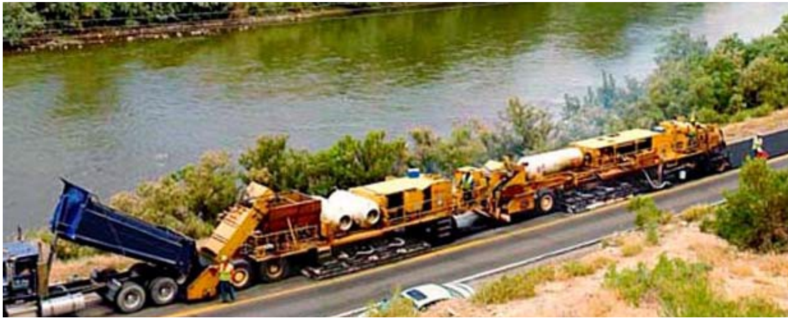
Figure 5-9 Surface Recycle Mix Placement*
