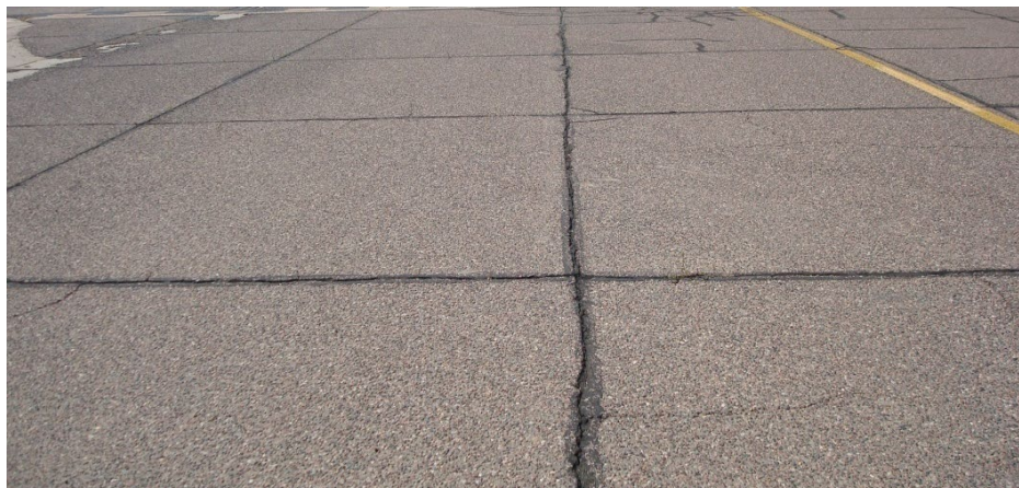
Figure 3-3 Reflective Cracking
