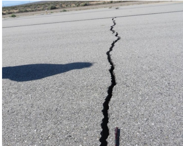
Figure 3-5 Transverse Cracking
