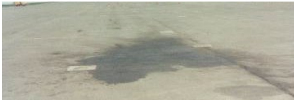
Figure 3-6 Fuel or Oil Spillage
