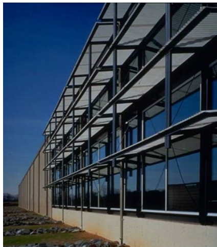
Figure A-4 Example of Architectural Shading Devices
