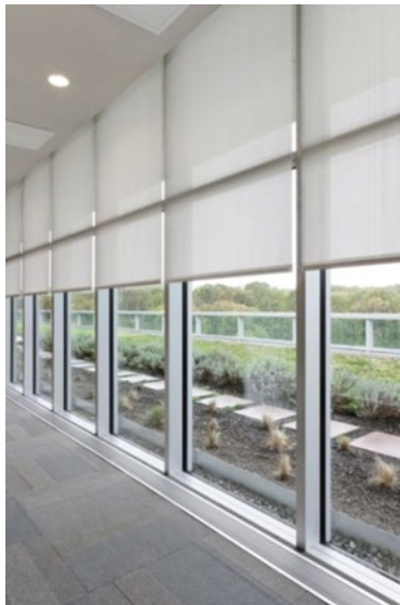
Figure A-12 Example of Solar-Adaptive Shading
