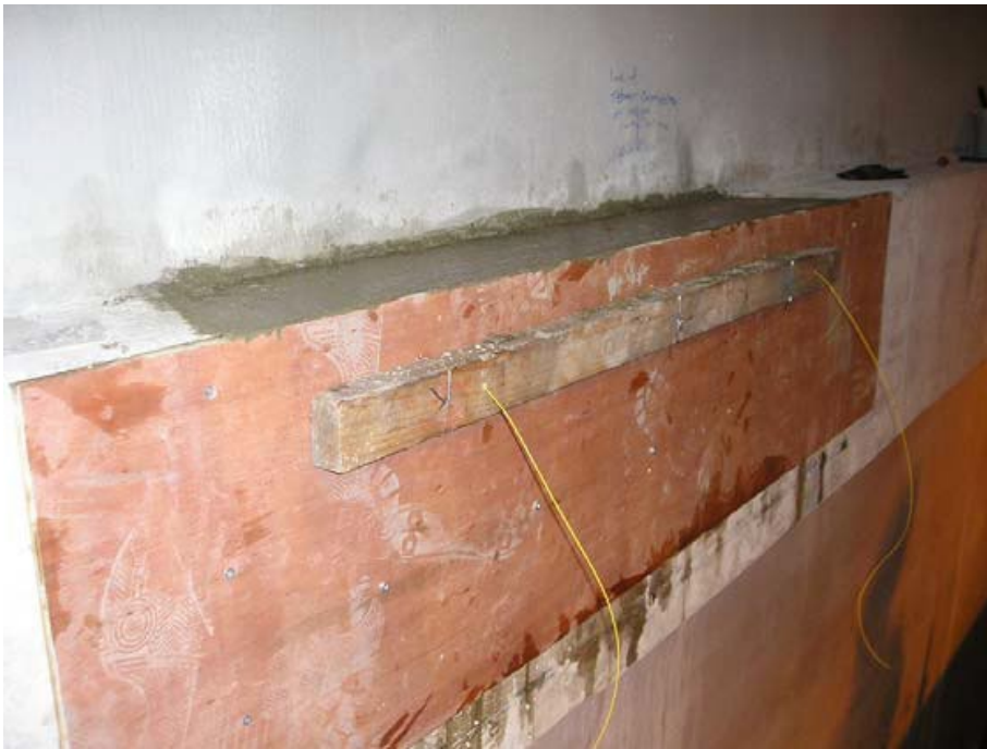
Figure B-11. An example of concrete repairs to ring girder side 1.
