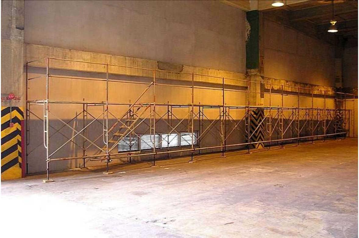
Figure B-1. Scaffolding in Building 306 Naha Military Port.
