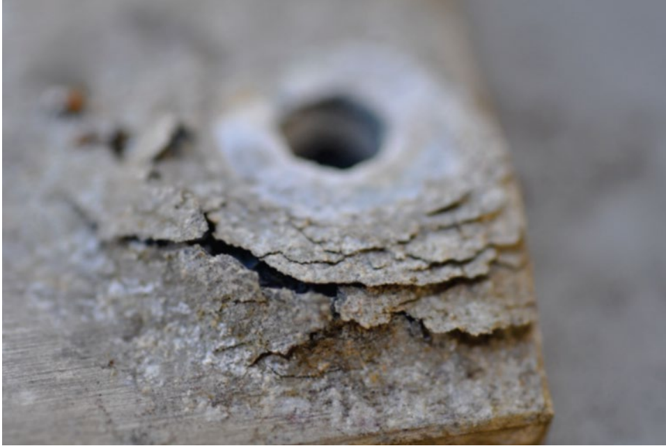
Figure 1-13. Exfoliation of a bare aluminum coupon after 24 months of exposure in a hot and humid climate.
