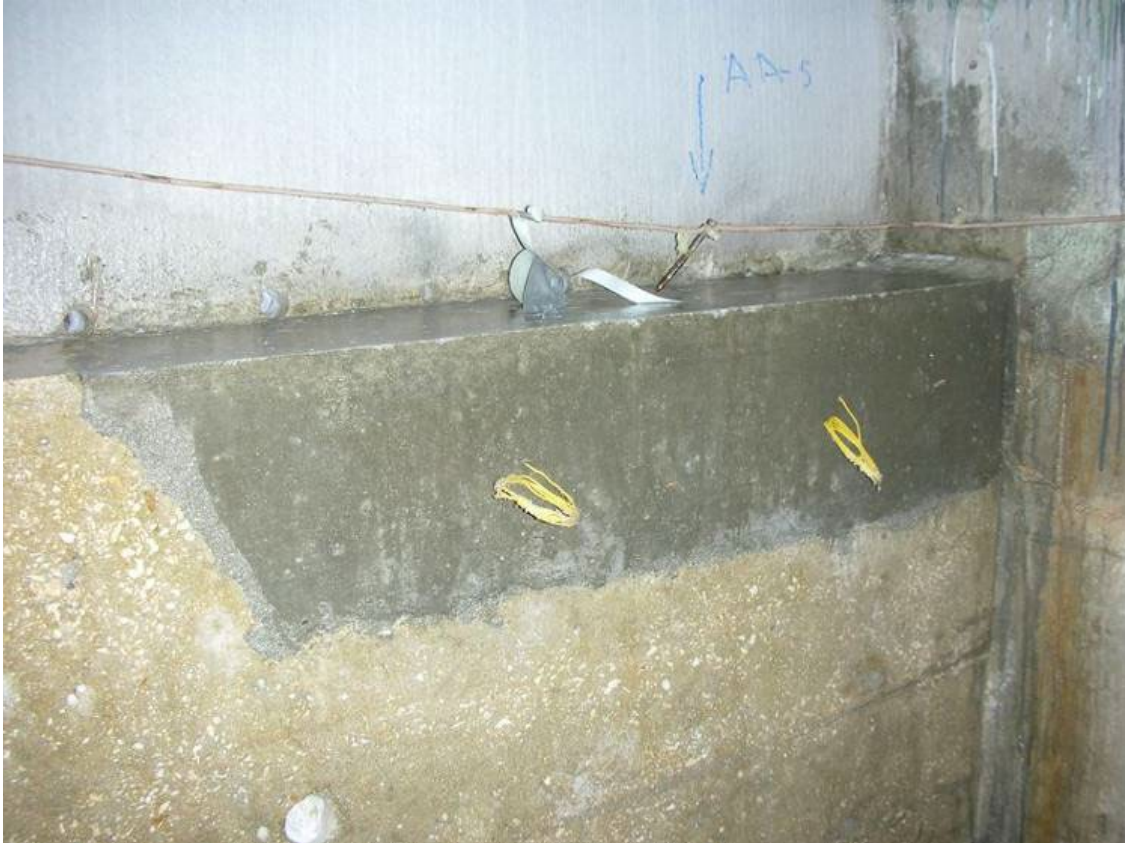
Figure B-13. Building 306, ring girder side 2 (NASA LGC).
