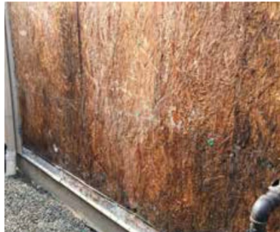
Figure 1-5. Example of saturated-oriented strand board (OSB) sheathing.
