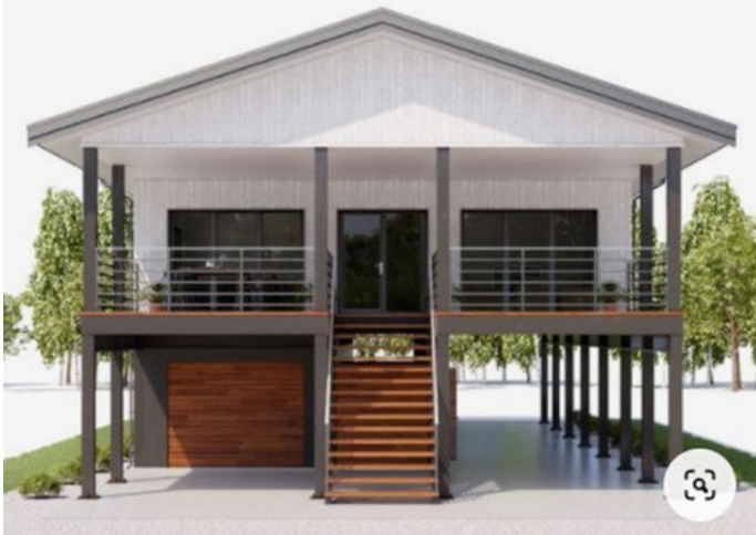
Figure 4-9. Raised construction is recommended where flooding is expected.
