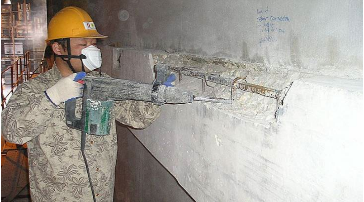
Figure B-4. Concrete repair.
