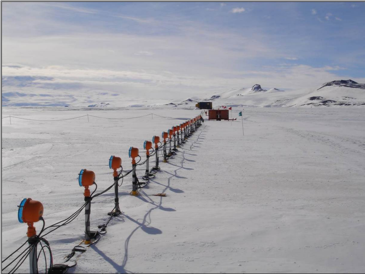
Figure 2-10 Typical Threshold Light Installation for Snow/Ice Airfields
