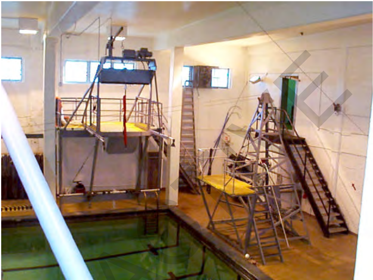
PHOTO 10 Hoist Rescue Trainer, Water Survival Pool
