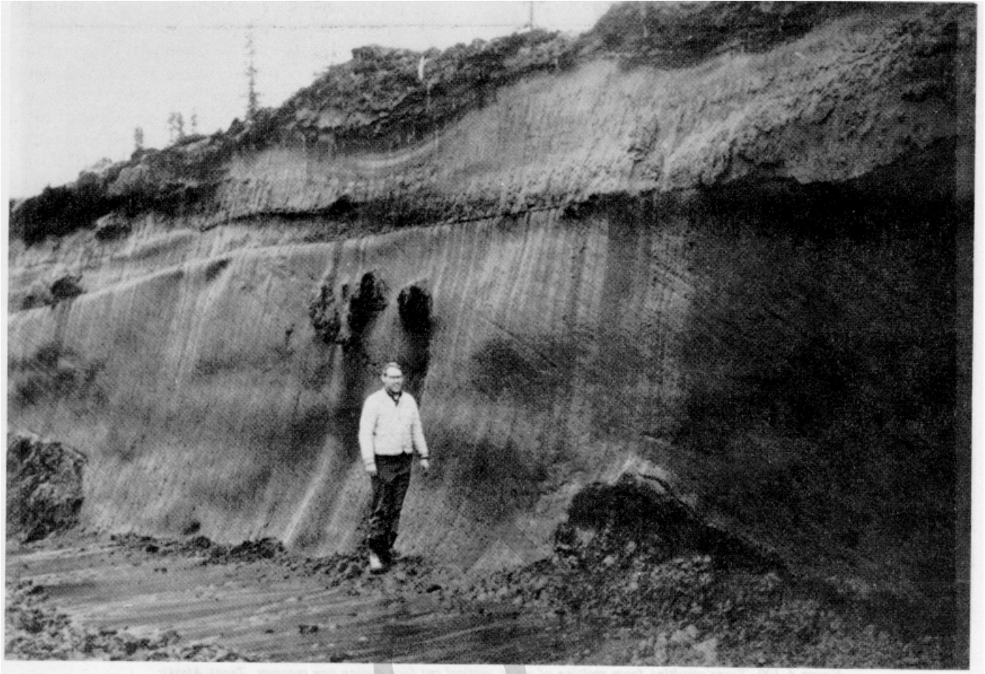
Figure 4-99. Ice exposed in vertical cut for Trans-Alaska Pipeline Access Road between Livengood and the Yukon River, Alaska, April 1970.
