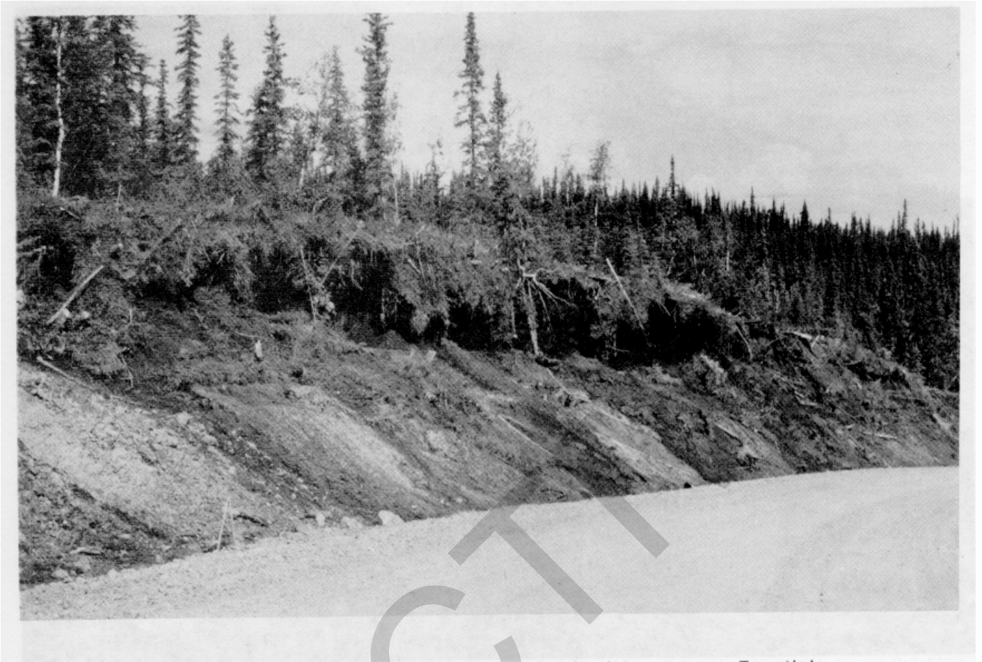
Figure 4-100. Slope resulting from melting of ice in vertical cut face during one summer, Trans-Alaska Pipeline Access Road between Livengood and the Yukon River, Alaska, August 1970.
