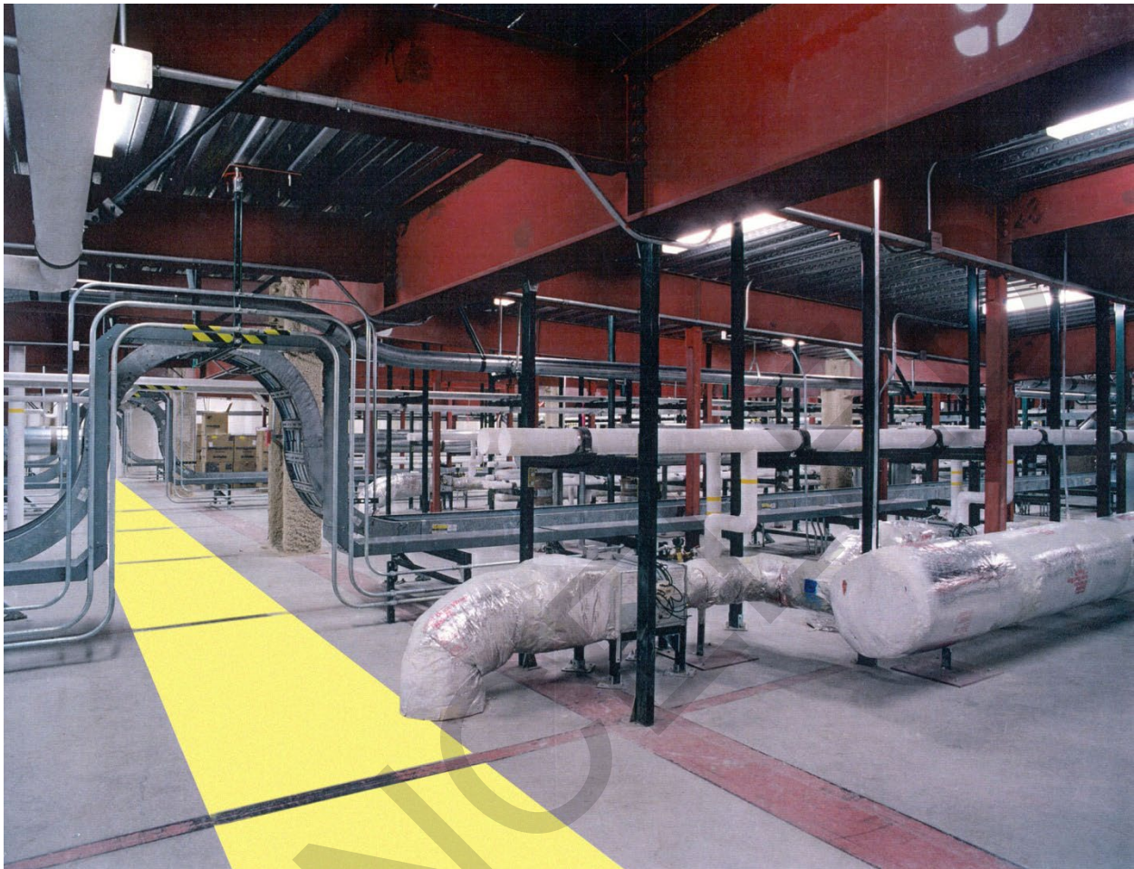
Figure E-3 Interstitial Access-Egress (Typical)
