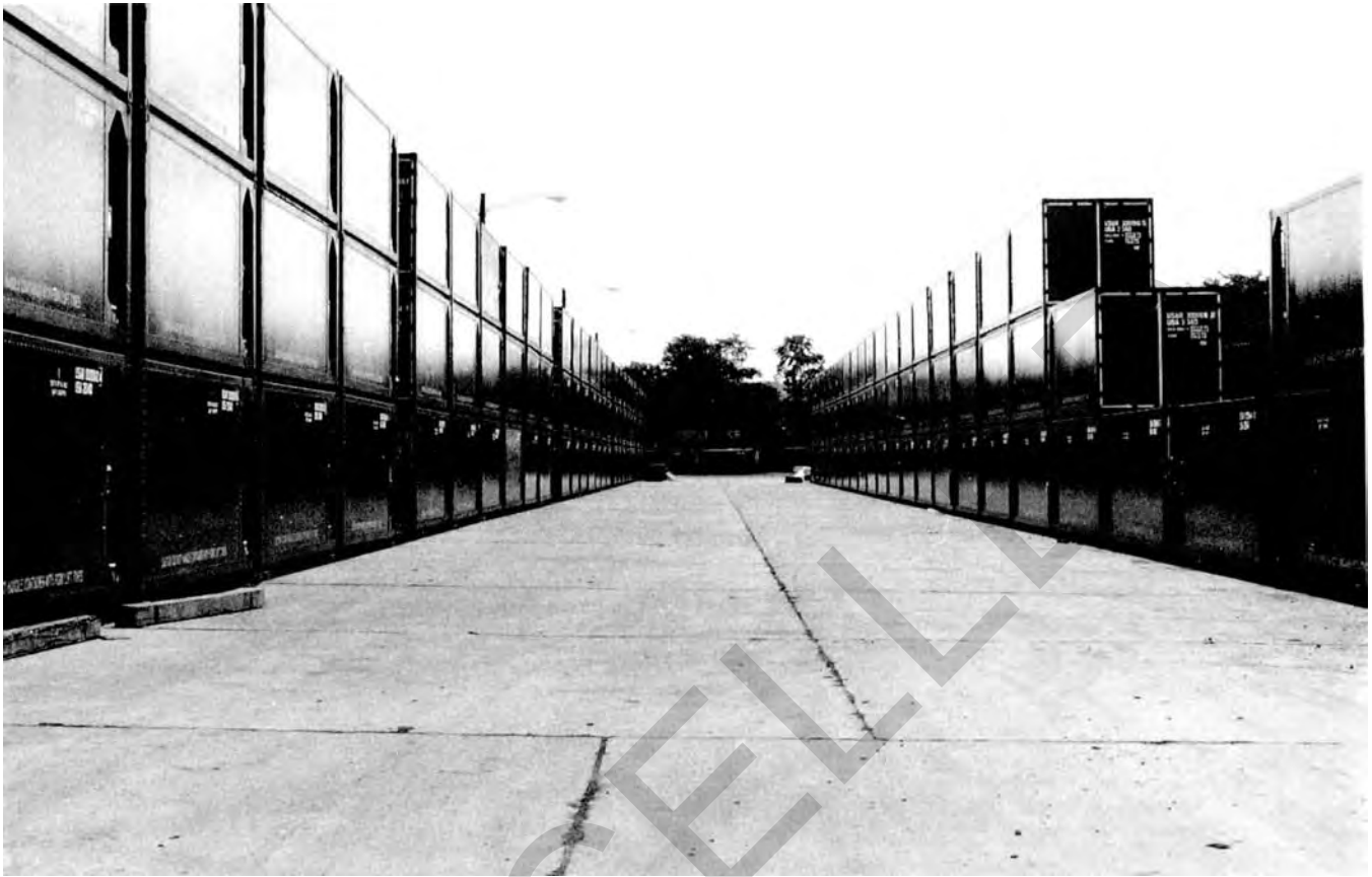
Figure 4-6. Containers stacked 3 high on concrete pavement.
