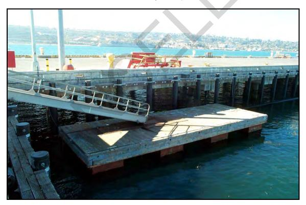
Figure 5-7 Plastic Fender Pile System.
