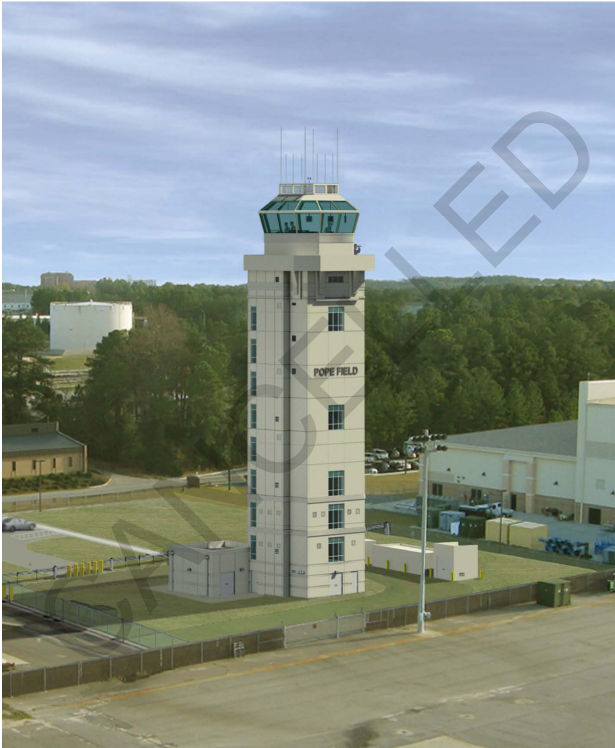
Figure 2-5 ATCT Functional Shaft without Support Building
