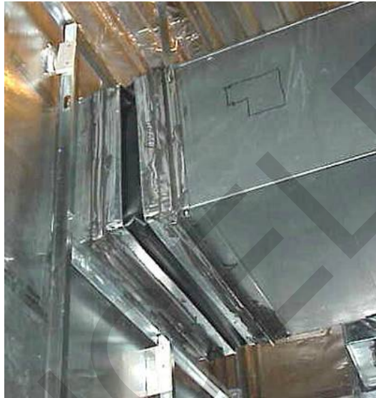
Figure 3-6 Duct Penetrations
