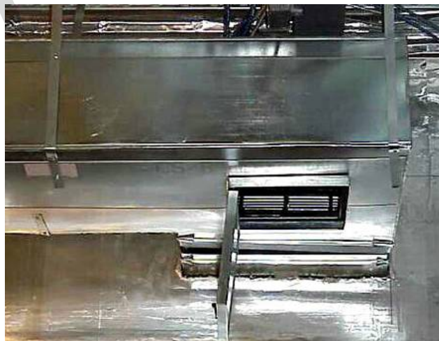
Figure 3-9 Access Port
