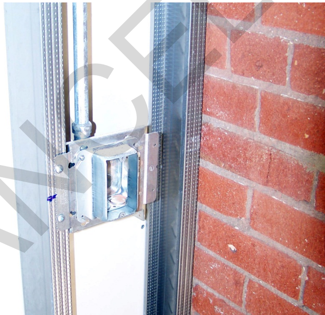
Figure 3-3 Furred Out Wall for Utilities
